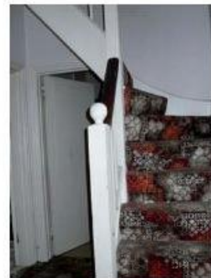
Secondary staircase up to second storey
