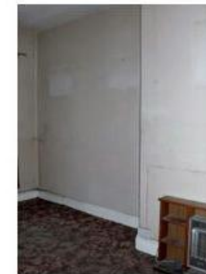
Room on western boundary with chimney breast and electric fire
