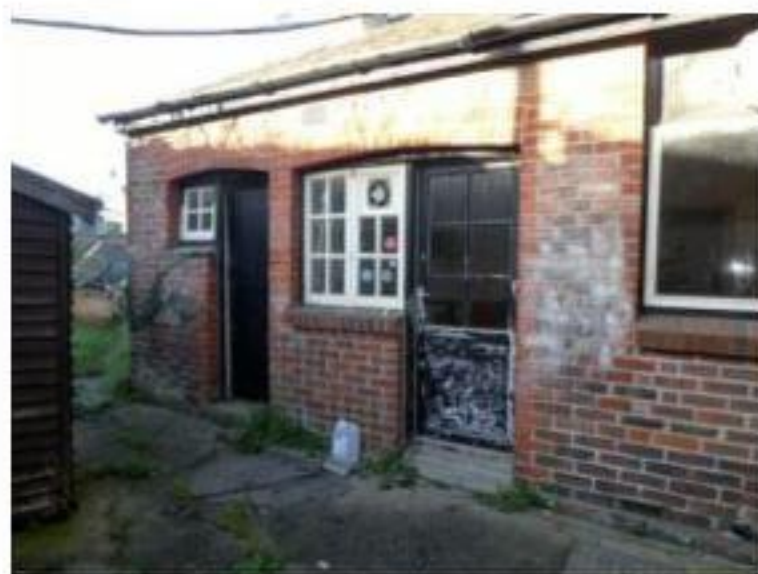
Looking towards single storey extension to rear of property
