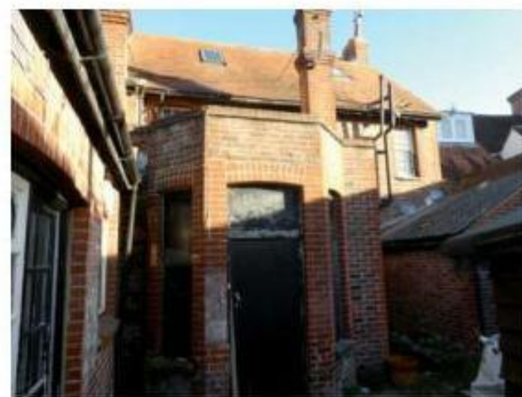
Looking towards rear elevation of property
