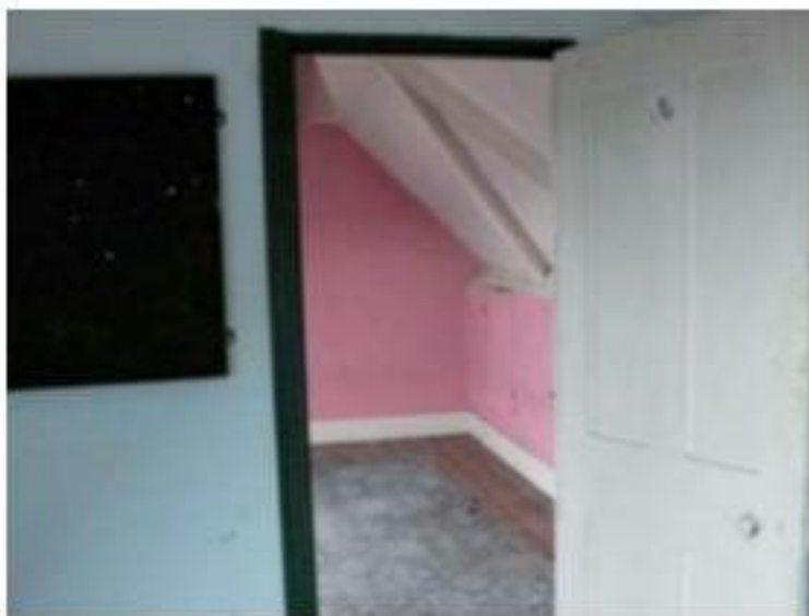
Second floor looking into west boundary room
