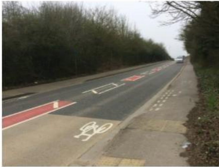
Photograph 1: Crookhorn Lane Infrastructure
