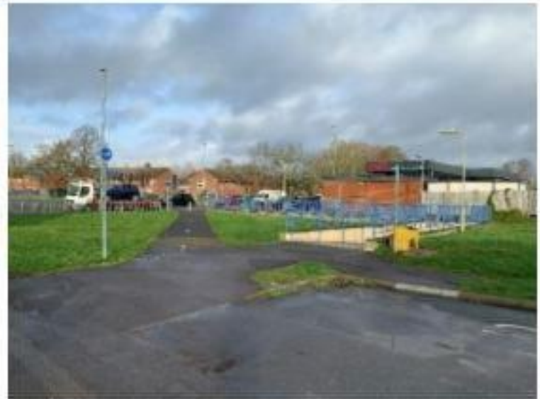
Photograph 2: Petersfield Road Subway
