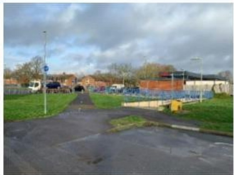
Photograph 4: Petersfield Road Subway
