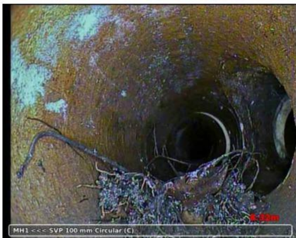
20191010-085806-snap0004.jpg, 00:01:48, 8.32 m Junction, at 03 o'clock, diameter: 100 mm
