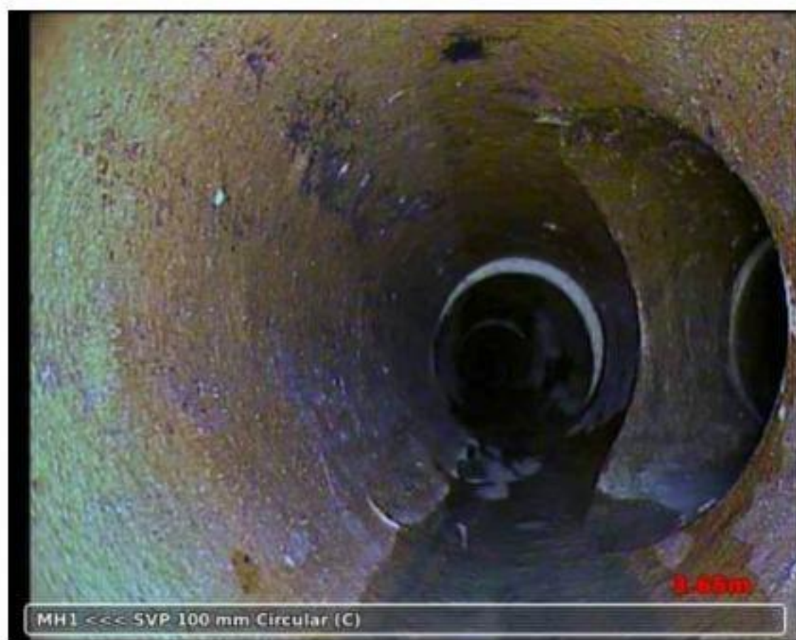
20191010-085806-snap0002.jpg, 00:00:34, 3.65 m Junction, at 03 o'clock, diameter: 100 mm
