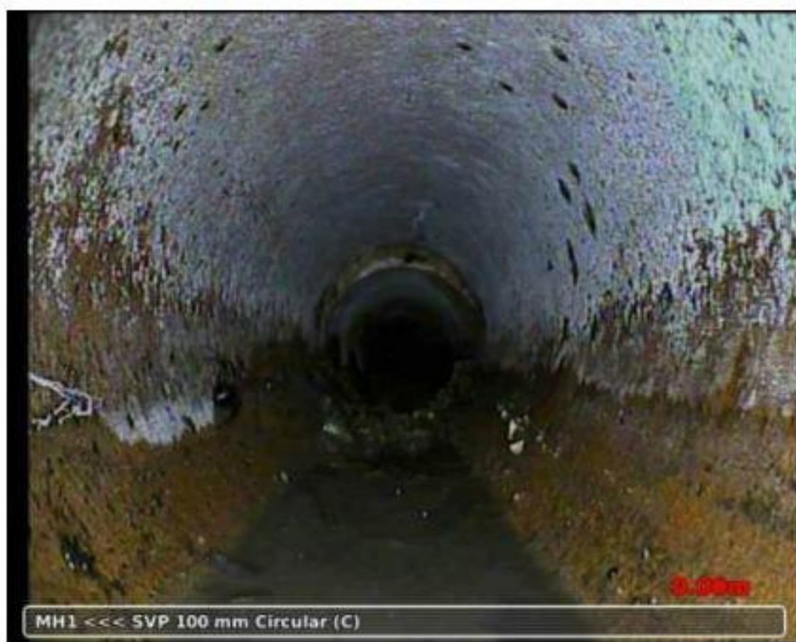
20191010-085806-snap0000.jpg, 00:00:02, 0.00 m Start node type, manhole, reference number: MH1
