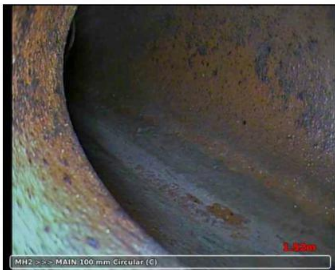
20191010-092247-snap0003.jpg, 00:01:10, 1.52 m Finish node type, major connection without manhole, reference number: MAIN
