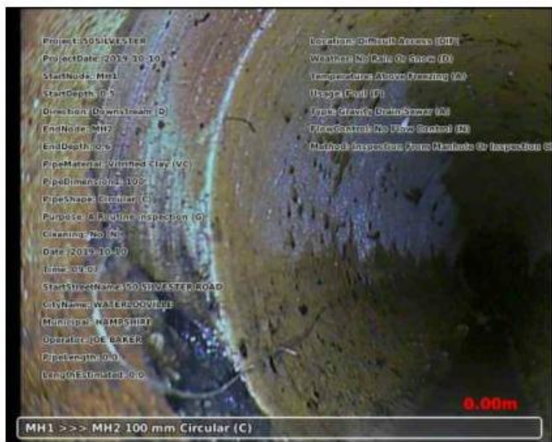
20191010-090906-snap0000.jpg, 00:00:01, 0.00 m Start node type, manhole, reference number: MH1
