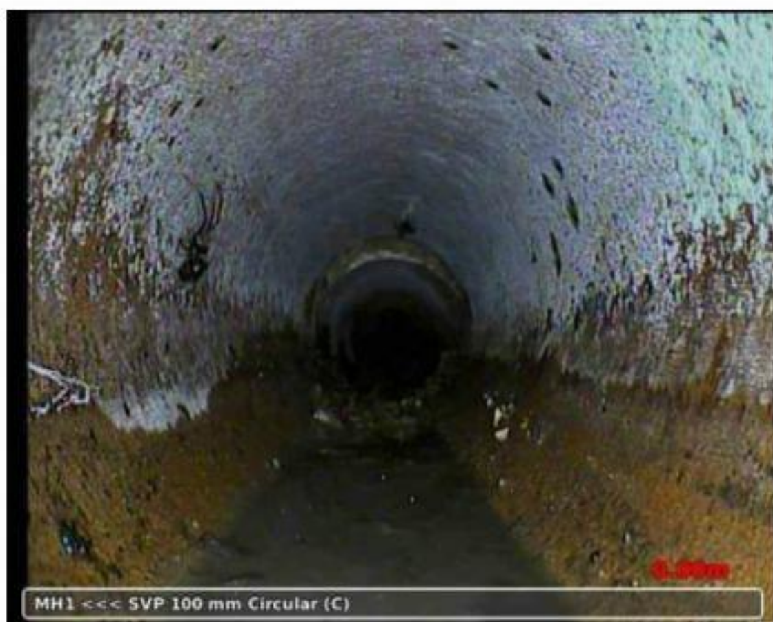
20191010-085806-snap0001.jpg, 00:00:06, 0.00 m Water level, 0 % of the vertical dimension
