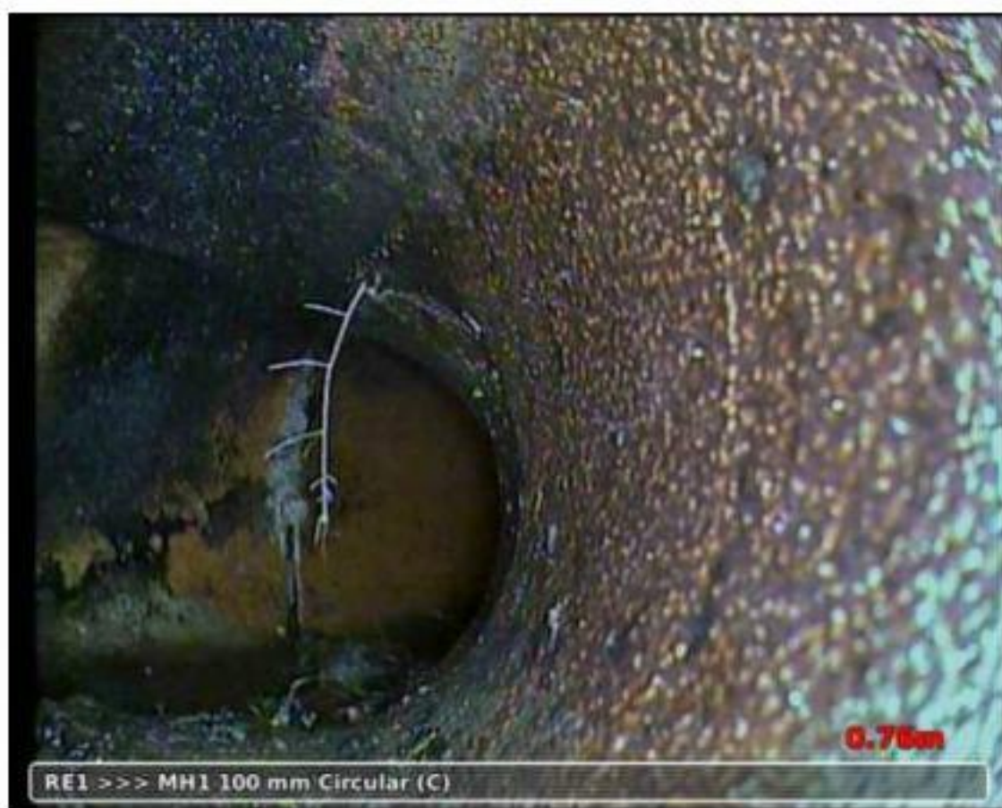
20191010-084757-snap0002.jpg, 00:00:30, 0.76 m Junction, at 09 o'clock, diameter: 100 mm
