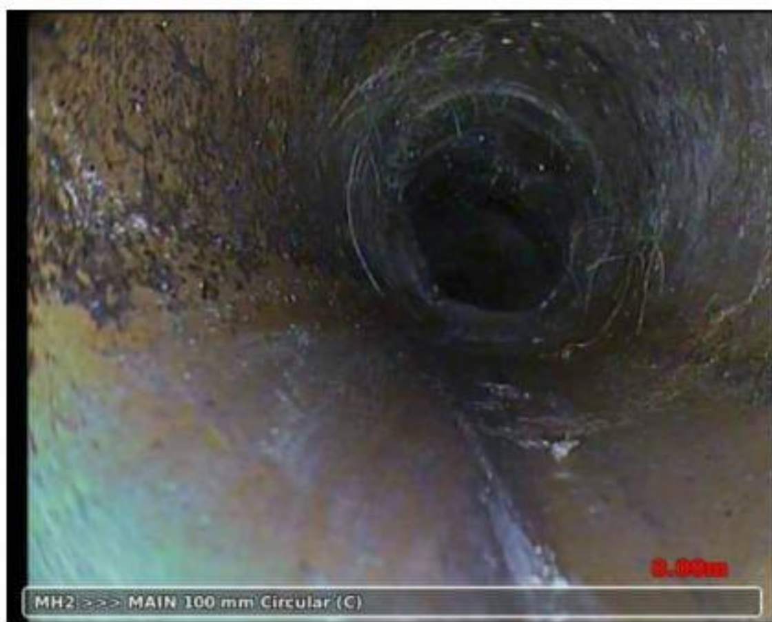
20191010-092247-snap0000.jpg, 00:00:08, 0.00 m Start node type, manhole, reference number: MH2
