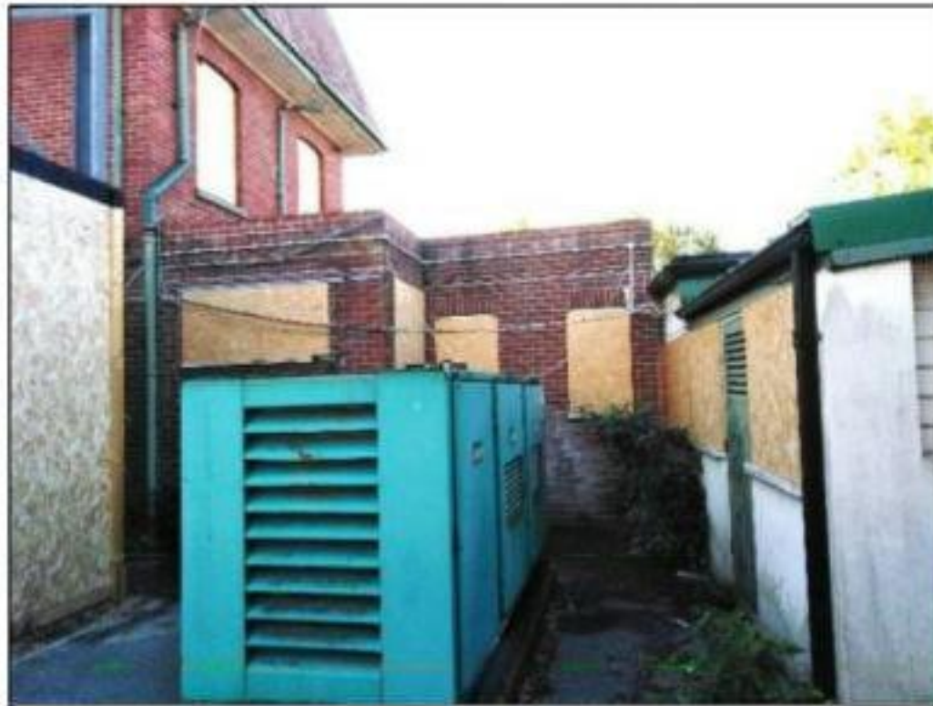
Photograph 9 Extensions to Building 1
