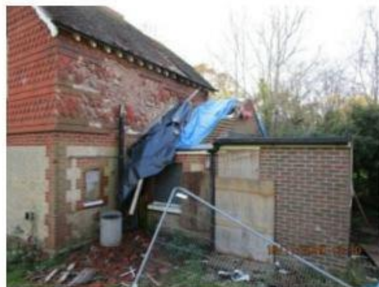
Damage to Tiling at The Gables
