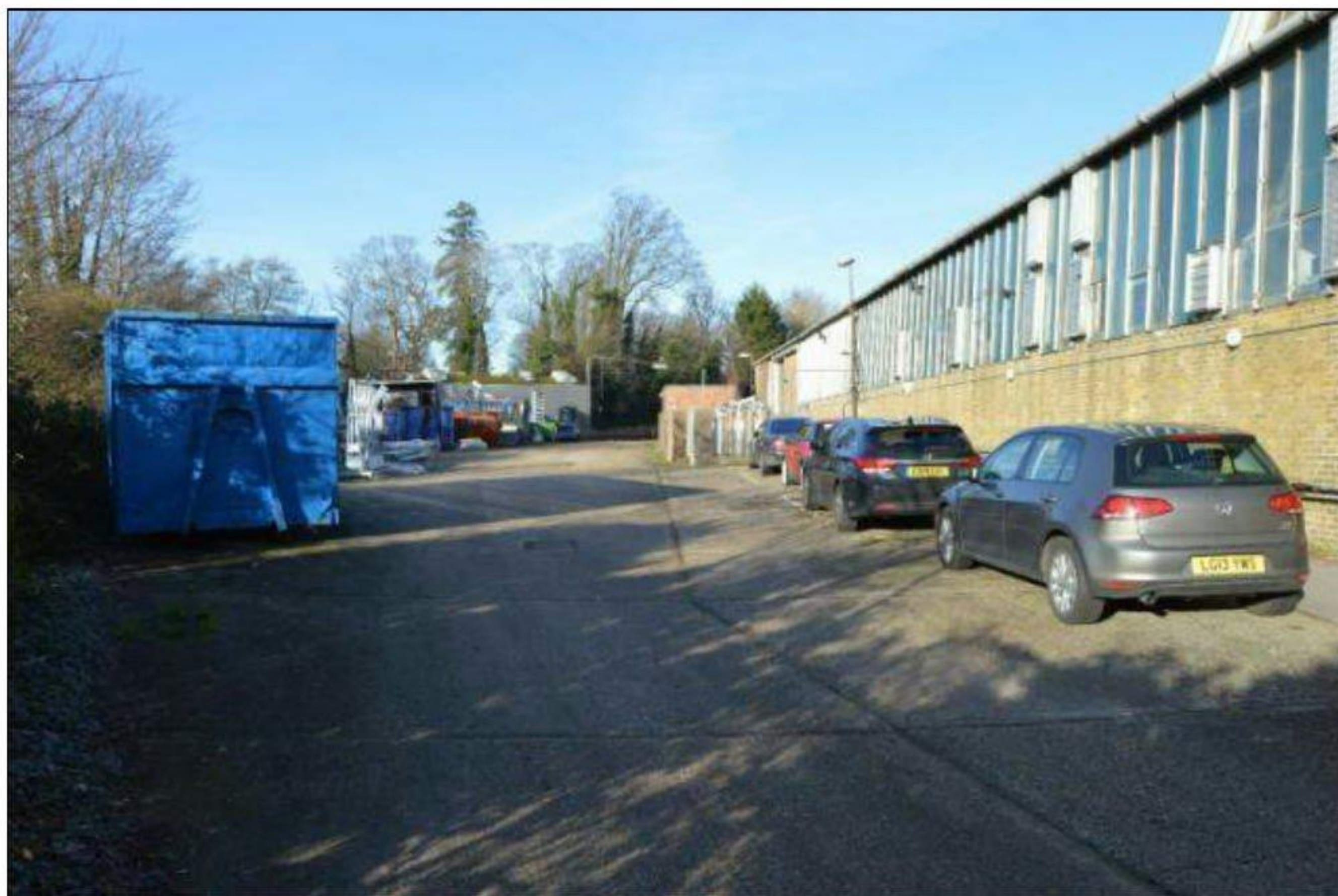
Photograph five: view along the southern perimeter of the site, facing northwest.
