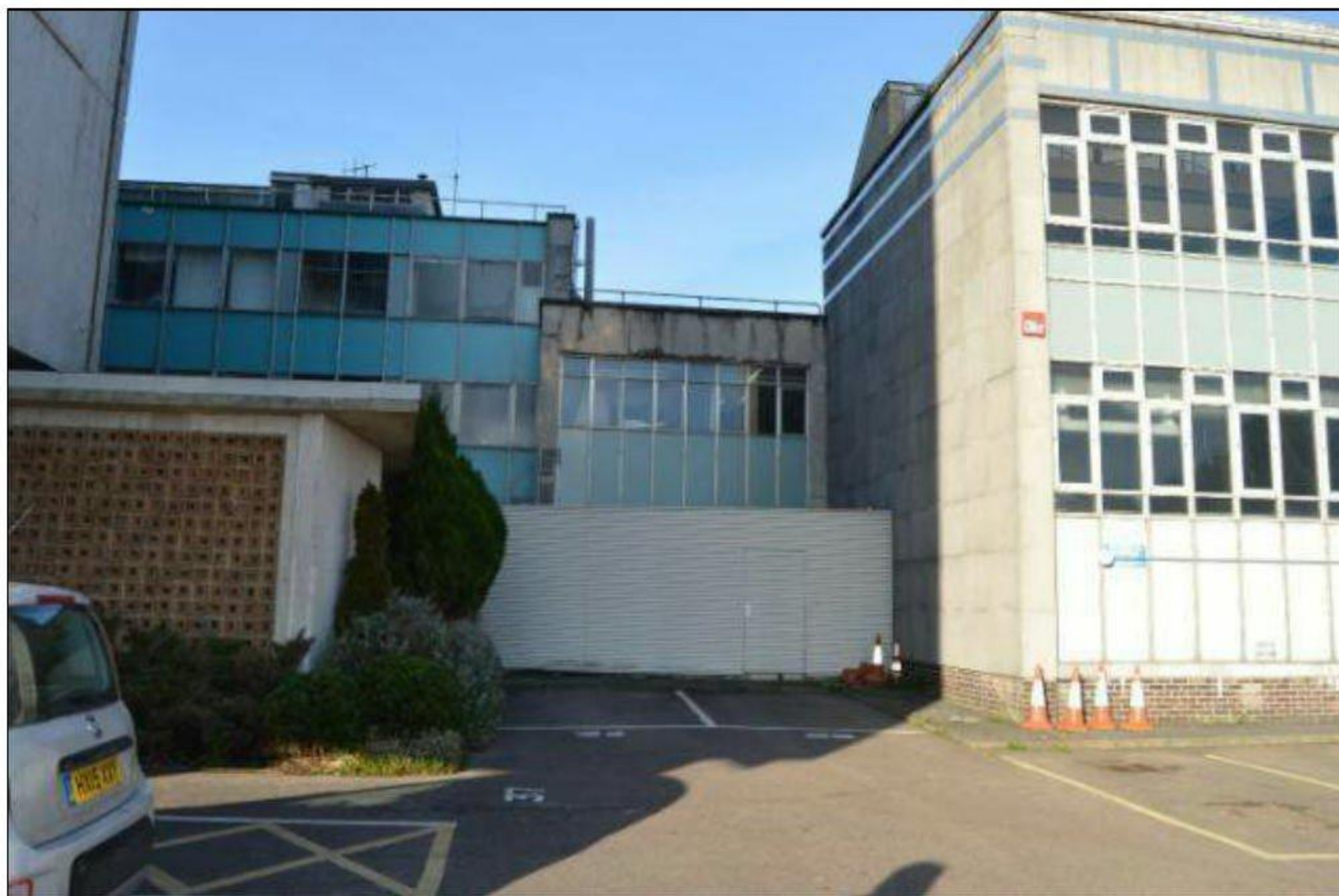
Photograph thirteen: possible access to a basement area between the main Colt office block and the R&D block, facing northwest.
