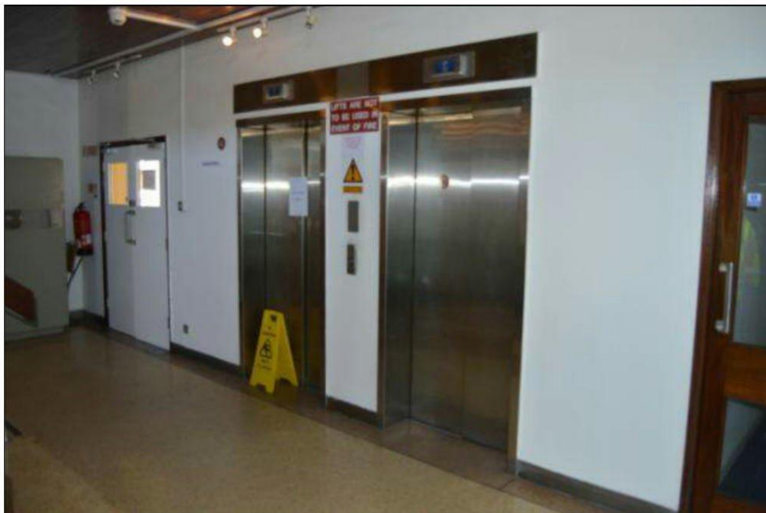
Photograph eleven: lift shaft in the ground floor of the Colt office block, facing southeast.
