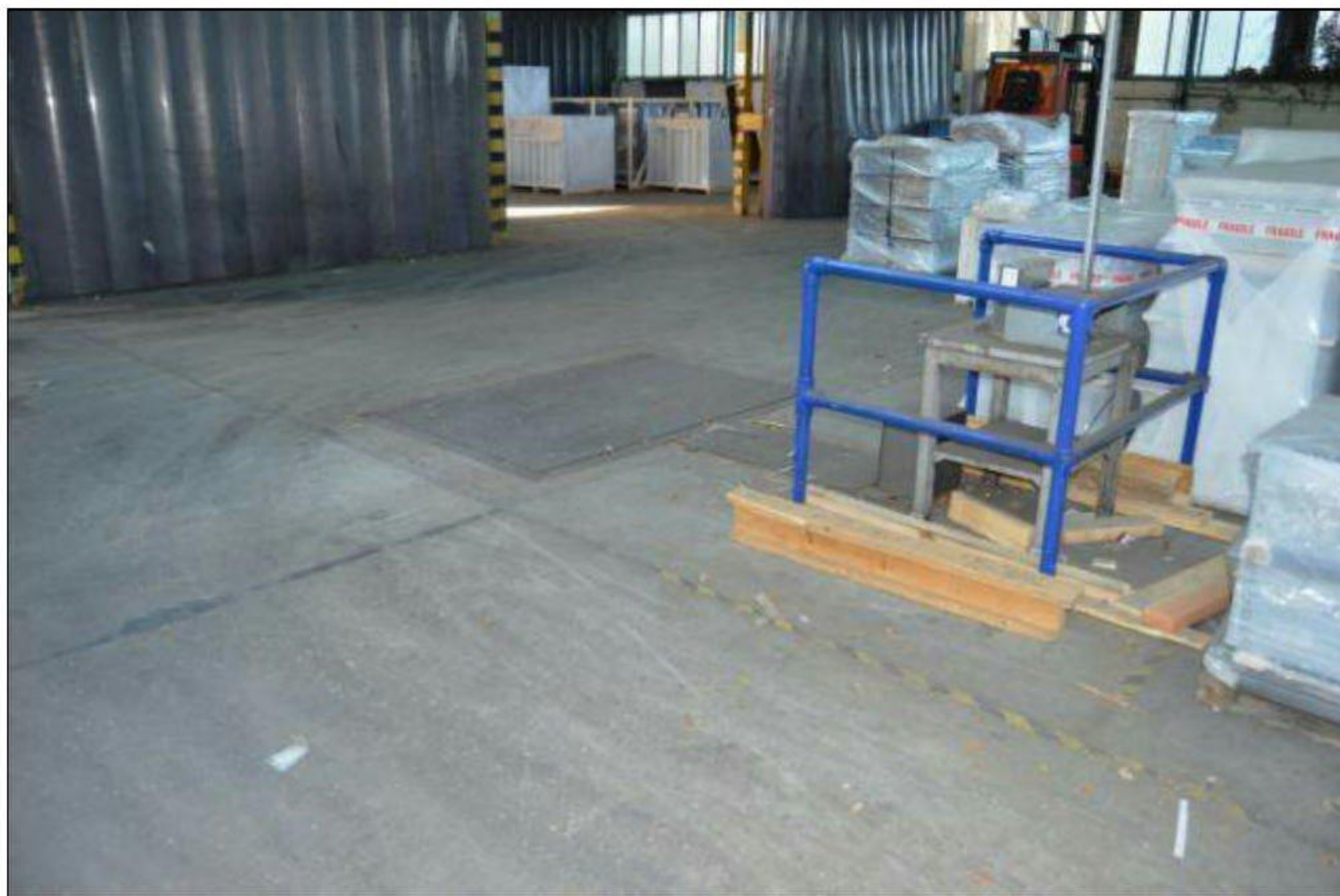
Photograph nine: floor covers associated with machinery in the factory complex, facing southwest.
