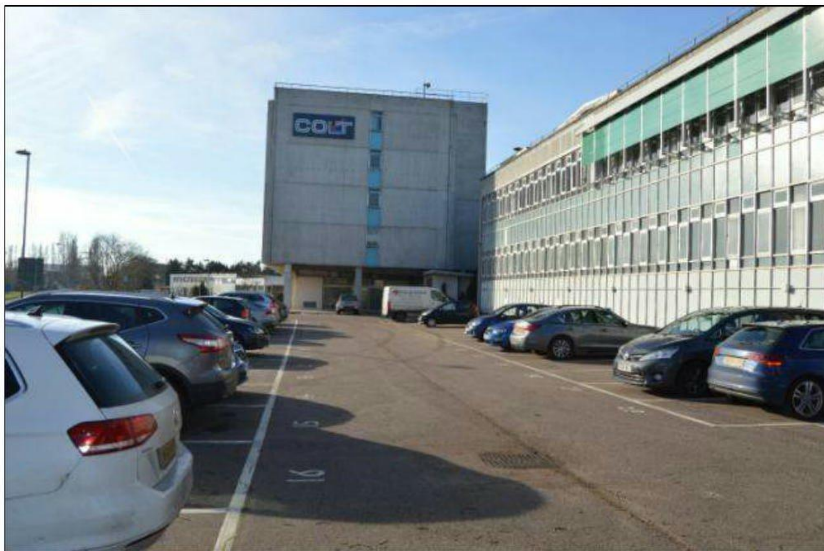
Photograph one: View of the Colt International office block from the northeast edge of the site, facing south.
