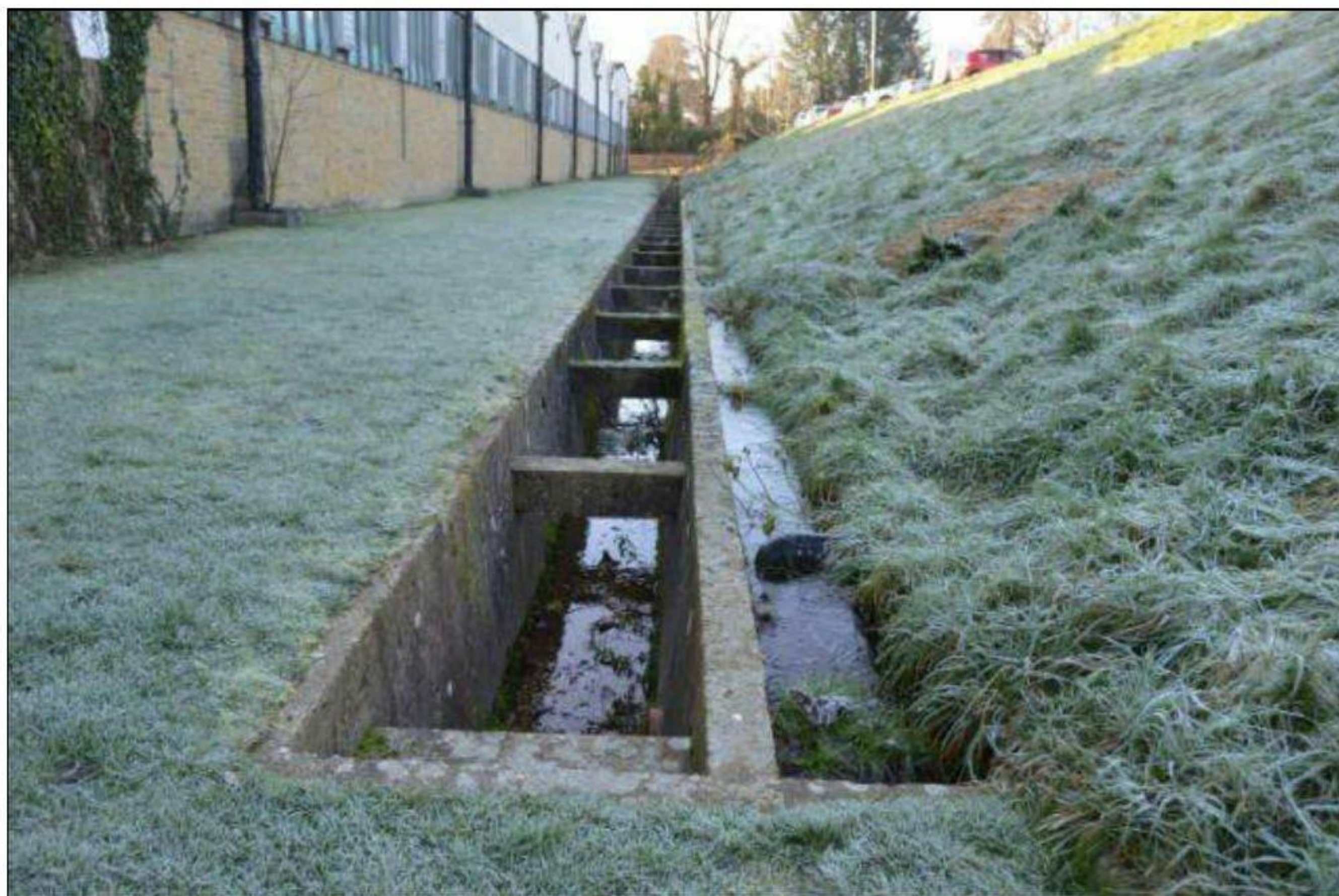
Photograph four: view along the monsoon drain at the base of the embankment, facing south.
