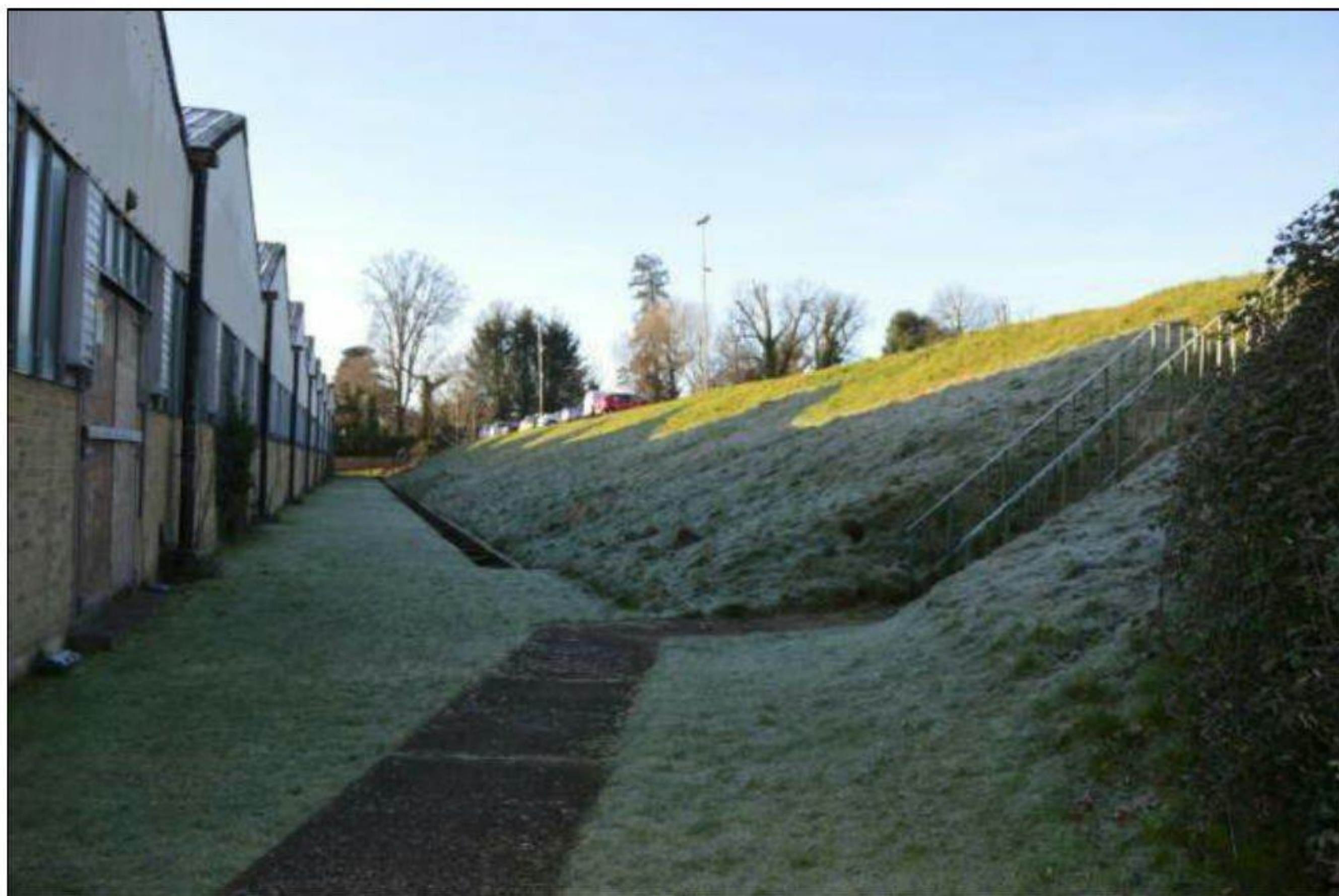
Photograph three: view of the embankment dividing the factory from the western car park, facing southwest.
