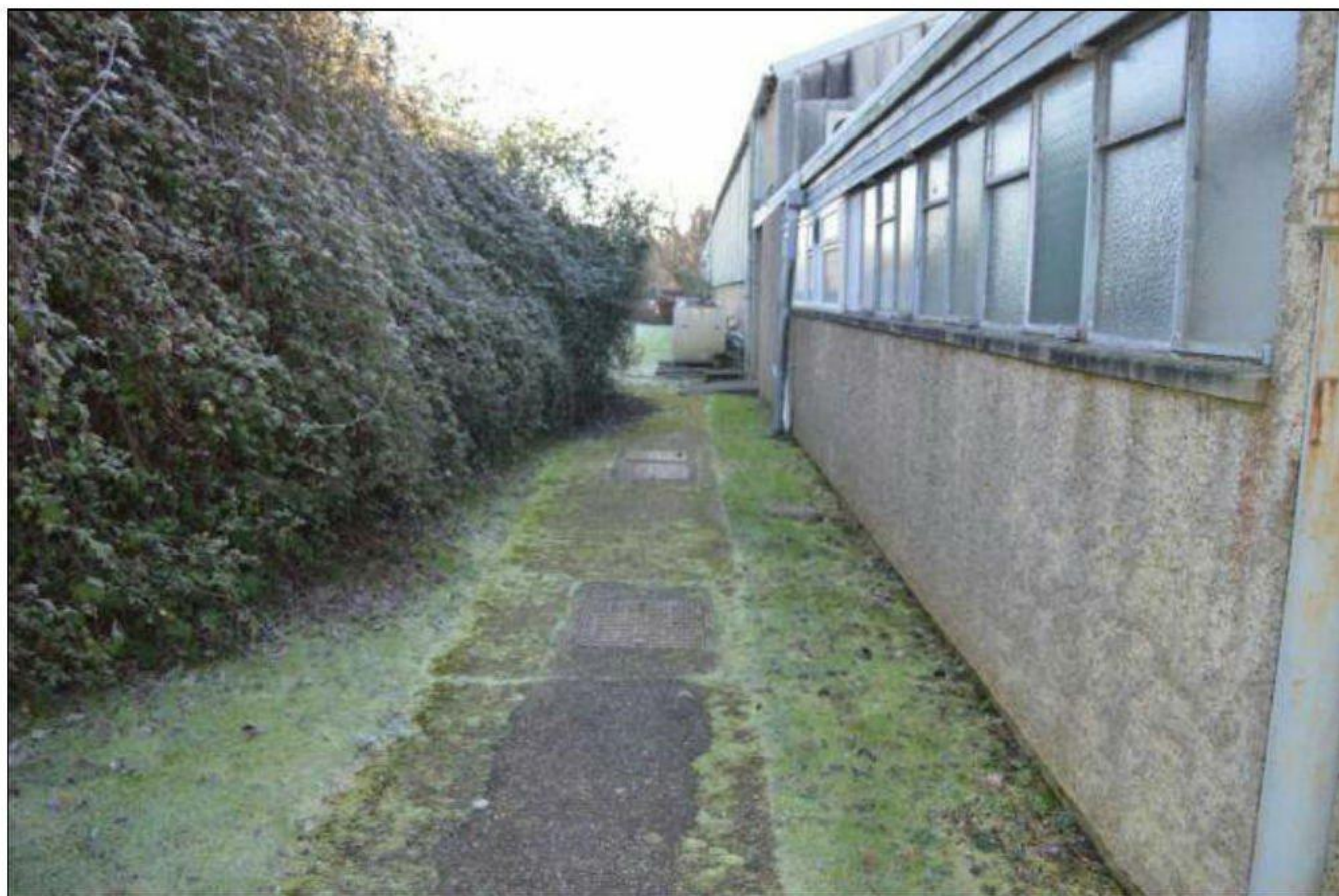
Photograph six: view along the northern perimeter of the site showing drainage covers, facing southeast.
