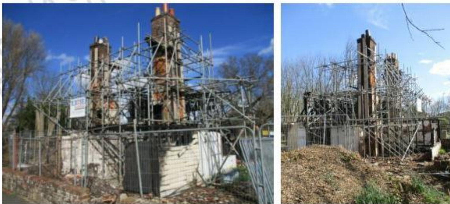
Figure 4 & 5 : Structural Scaffolding (March 2019)
