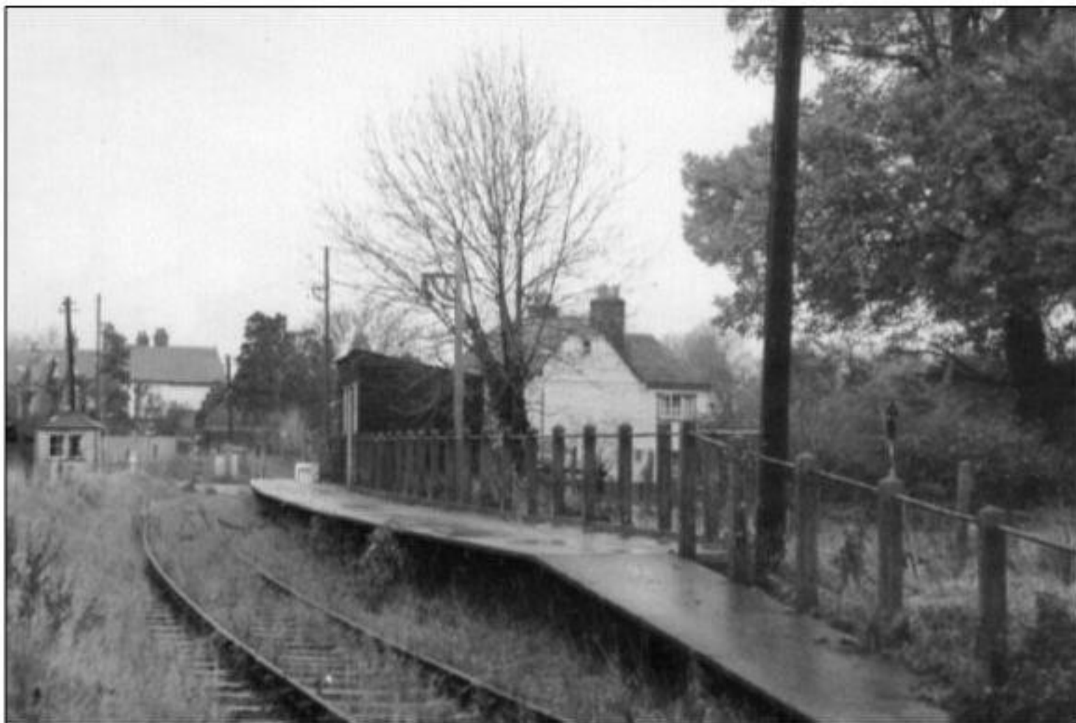
Figure 17: Post 1963 image of 'Langston' Halt/Station after the Hayling Railway closed, showing the cottages in the background (Whitwell, N, n.d)
