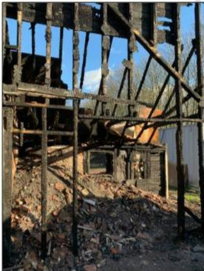
Figure 23: The cottages after the devastating fire (Jan, 2019)
