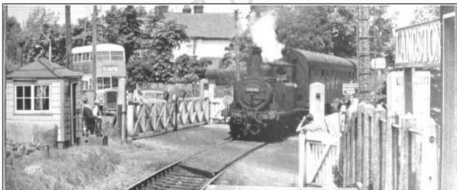
Figure 16: Langstone Level Crossing (Griffiths, G, n.d)
