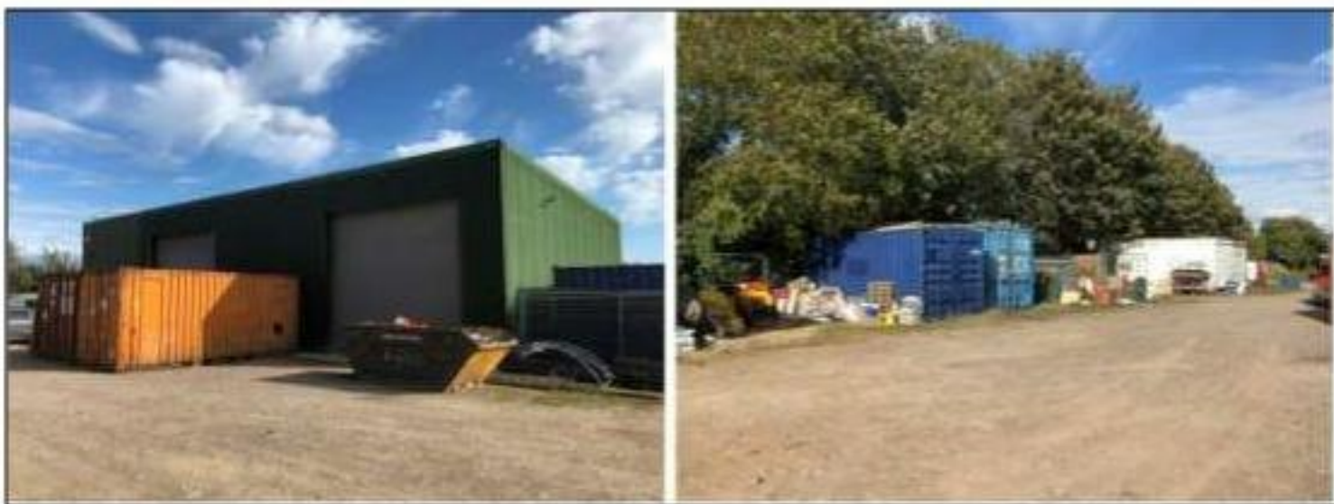
Figure 1. Commercial Building at 15 Lower Road, Bedhampton.
