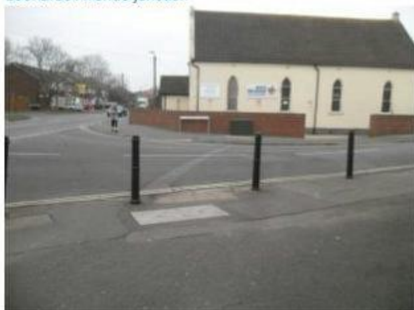
Photo 3.5: Dropped kerbs/tactile paving, Elm Grove/St Leonards Avenue junction
