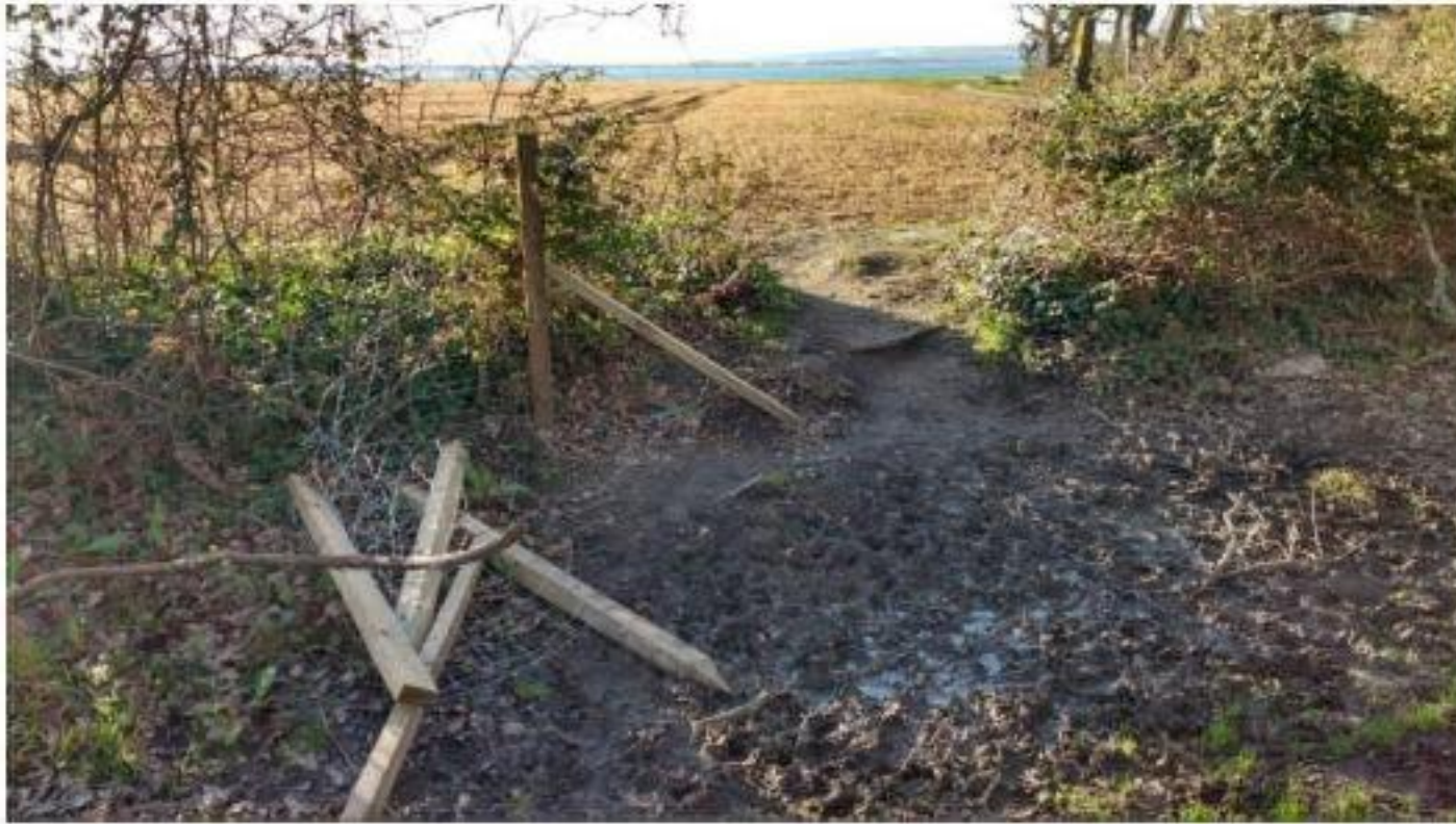
Photo i: Broken down fencing, recently installed by Barratt Homes after it was shown that they had not carried out agreed mitigation for the The Oysters Development. It is clearly not robust enough to keep dog walkers from walking into field at north end of H34C looking west over destroyed crops. (24 th March 2019)
