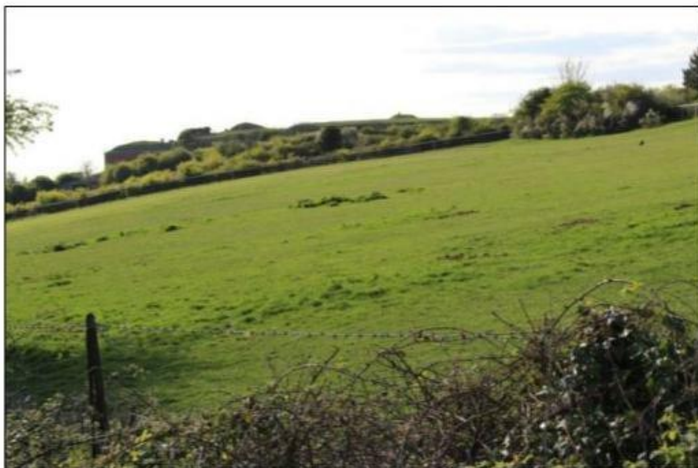
Figure 26. View of Fort Purbrook from its east side show how its southern elevation is more prominent than its northern side due to how it was constructed partially within the slope of the hill. This view gives a clear understanding of how the fort was not intended to be a dominant feature in views from the north.
