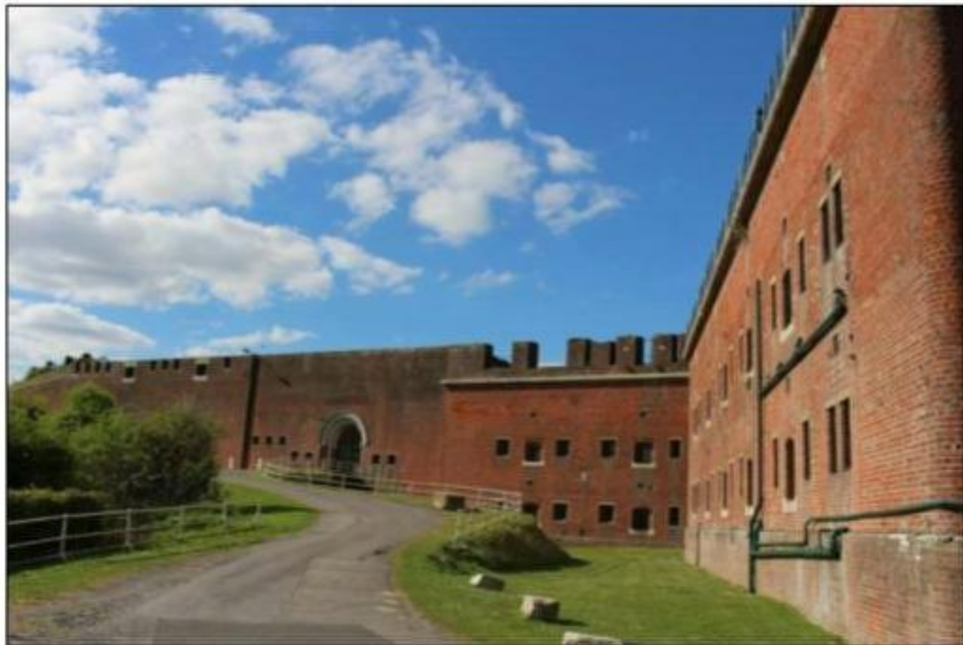
Figure 13: View along the western side of the south elevation of Fort Purbrook.
