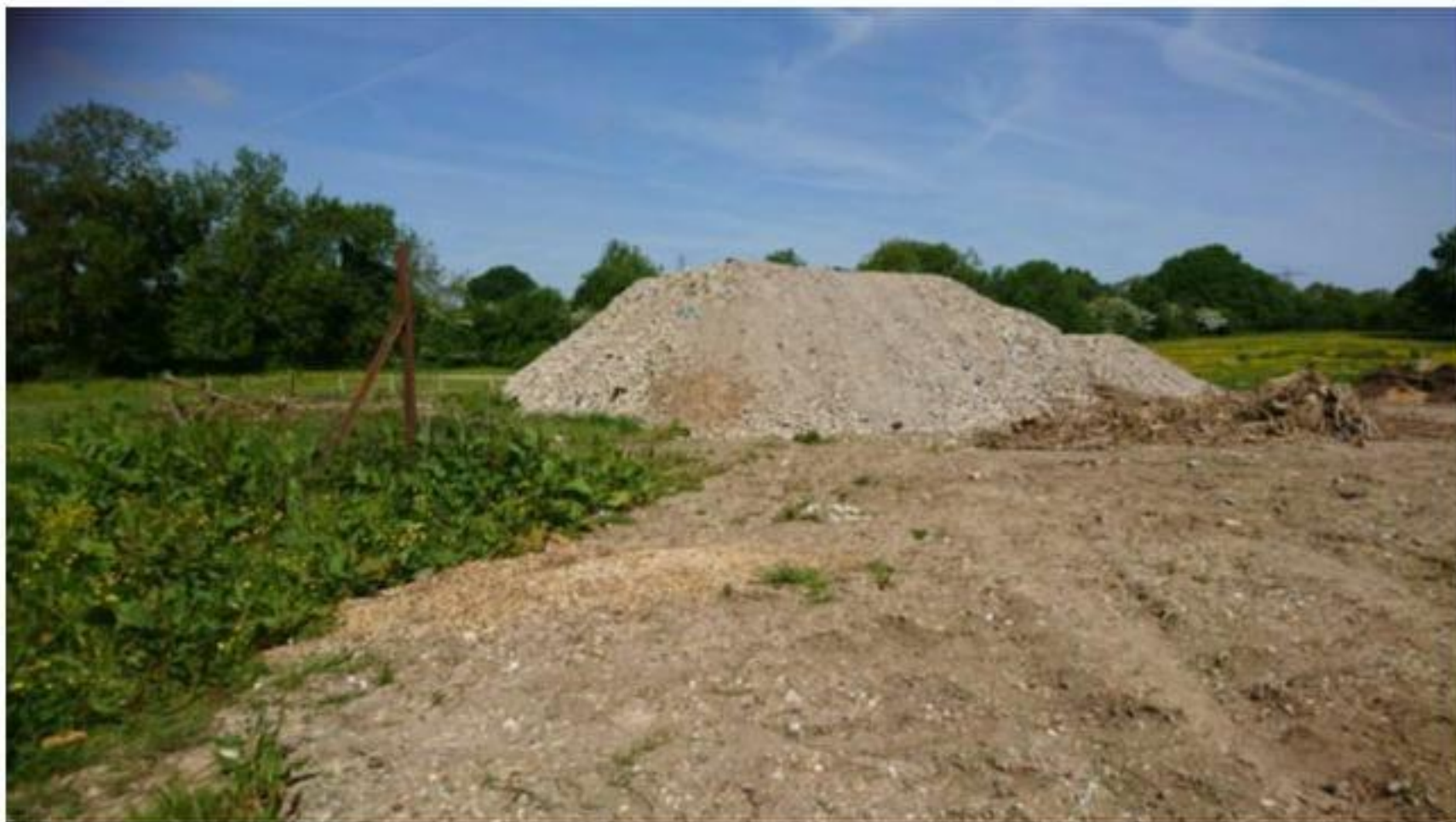
Plate 8 View north west of crushed concrete stockpile
