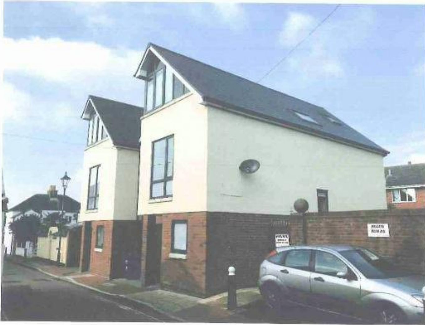
Figure 5: Existing Dwelling as seen from Nils Street (East)
