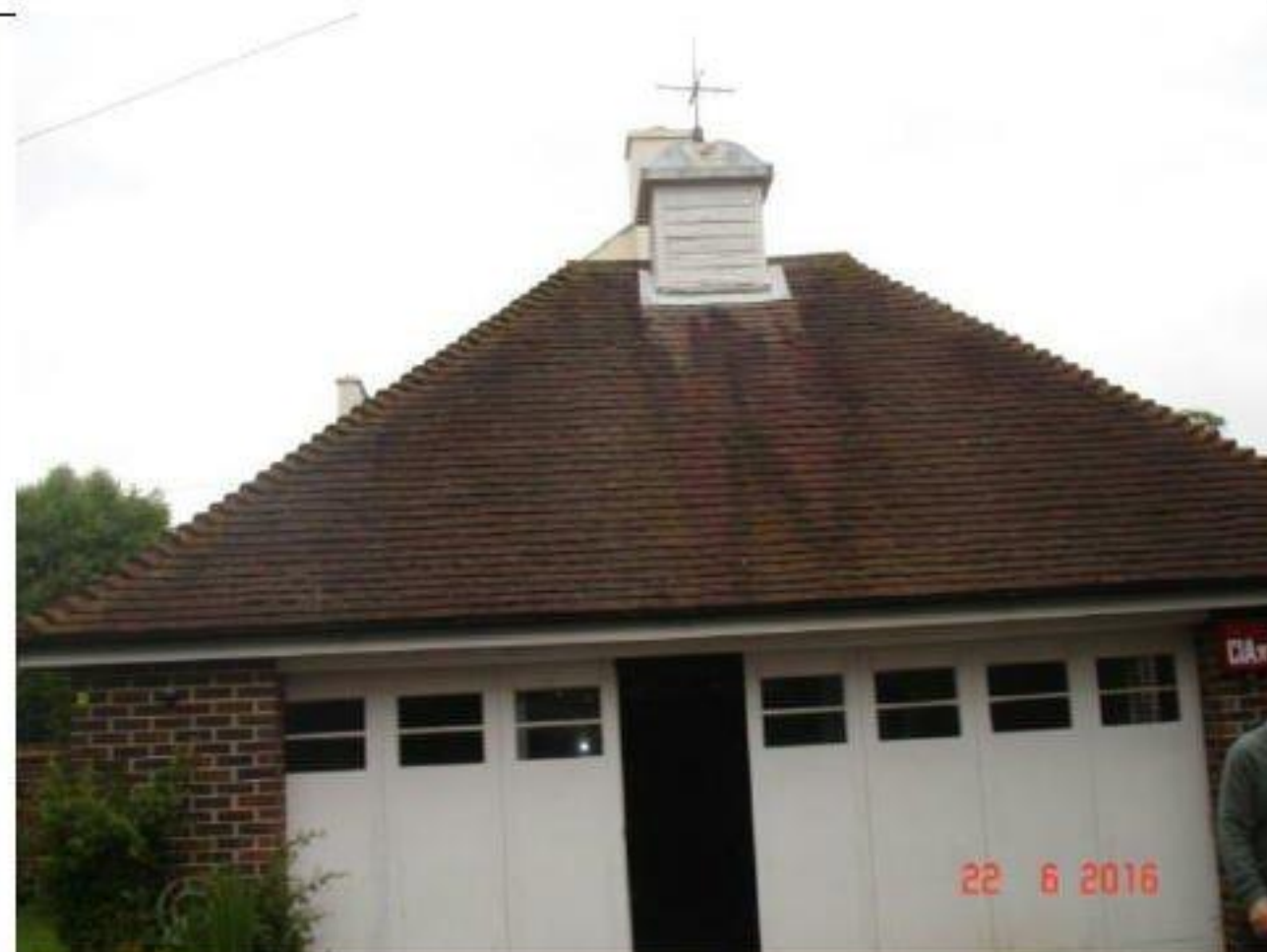
Photograph 2: View of the southern aspect of one of the detached double garages.
