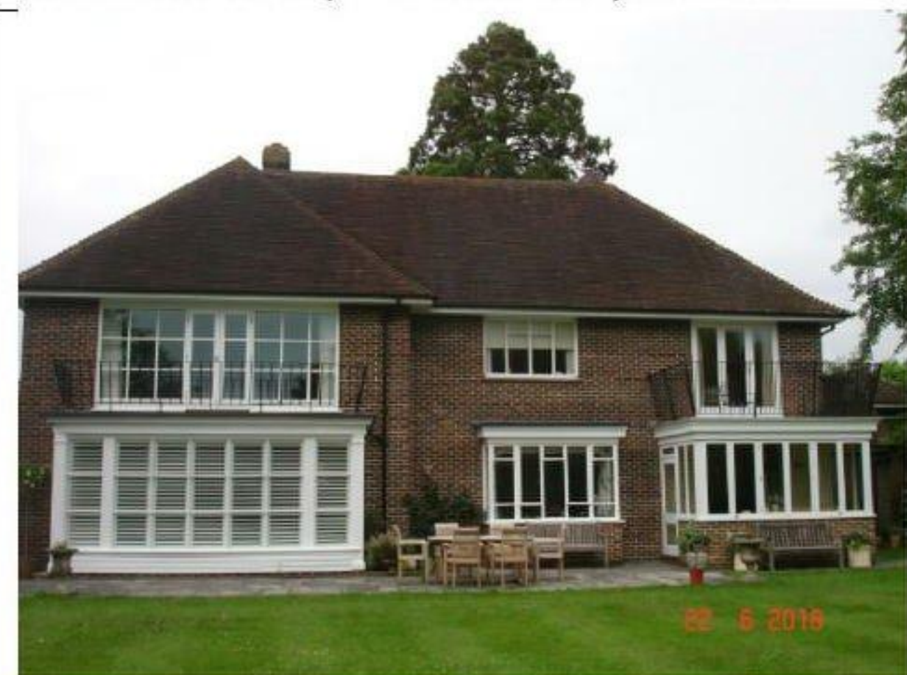
Photograph 1: View of southern aspect of residential building.
