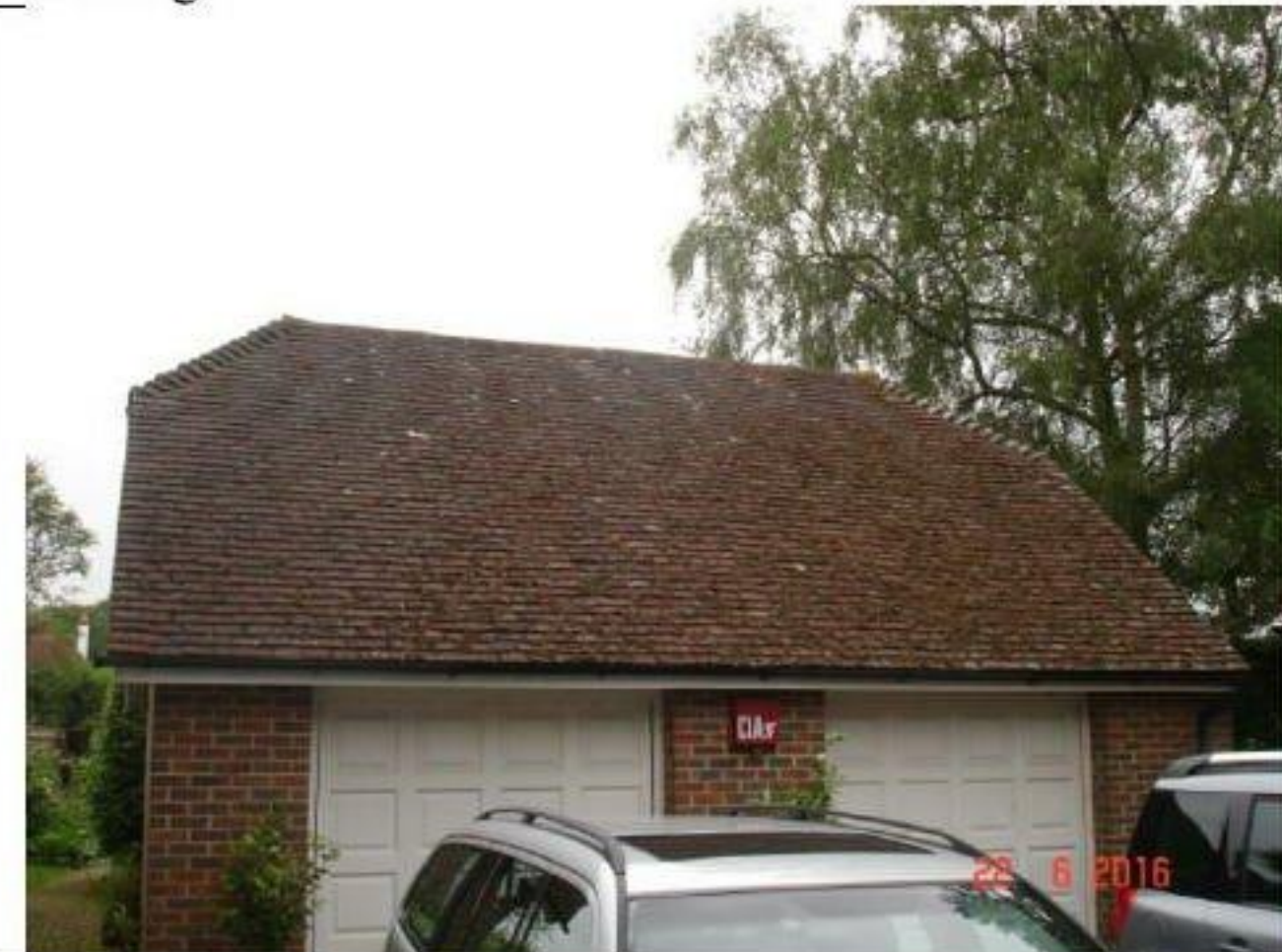
Photograph 3: View of the western aspect of the second detached garage.
