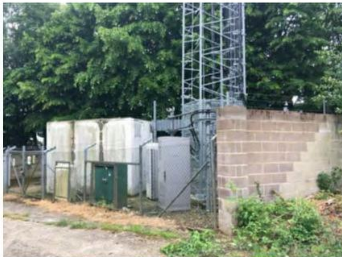
Photograph 4 - Radio mast and substation
