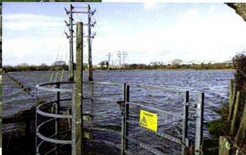
Photograph D facing east showing combined fluvial and tidal flooding. The River Lavant has over spilled into Southmoor adjacent to Mill Lane south of the weirs. The sea wall has been overtopped.
