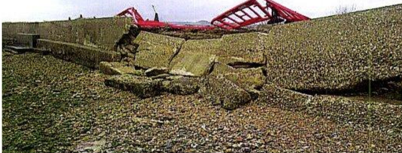
Figure 1-2: Existing condition of the sea wall
