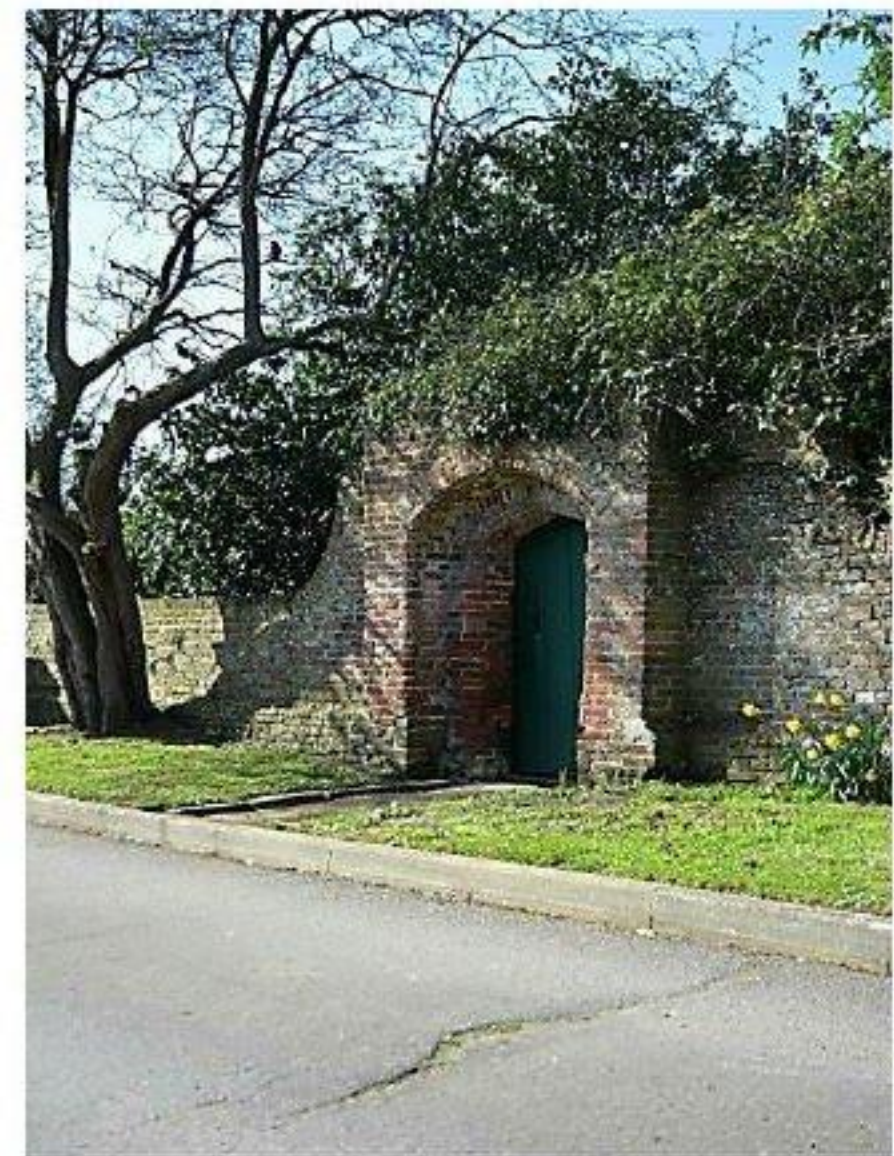
Access permits only light vehicular traffic
