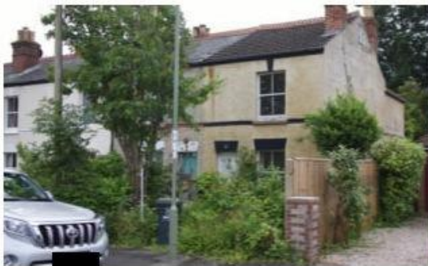
Fig (4) Repositioning of street-light
