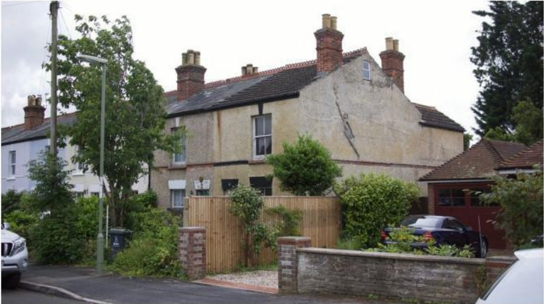
Fig (1) Properties viewed from King's Road
