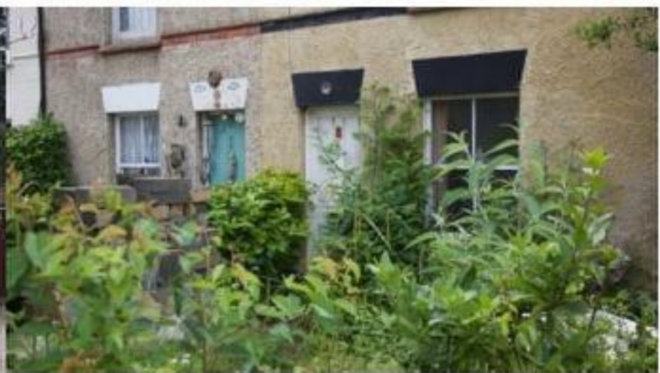
Fig (5) Present condition of dwellings (externally & internally)
