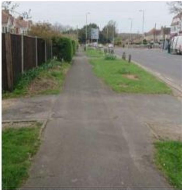
Photograph 48: Footway Conditions along Bedhampton Road
