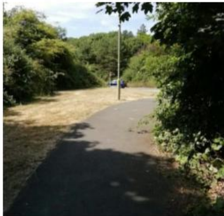
Photograph 52: Footway/cycleway from Lower Road to Rusty Cutter Roundabout
