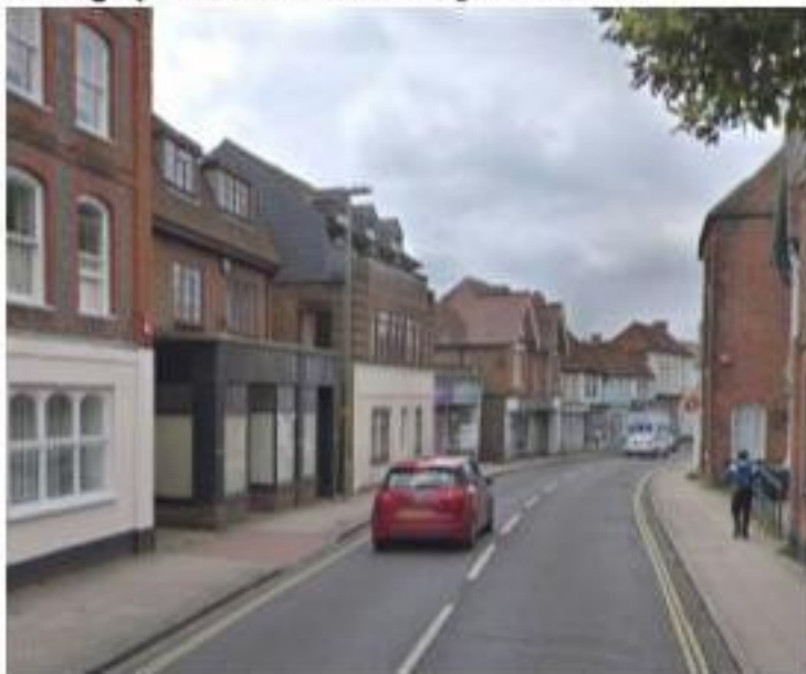
Photograph 63: Conditions along East Street
