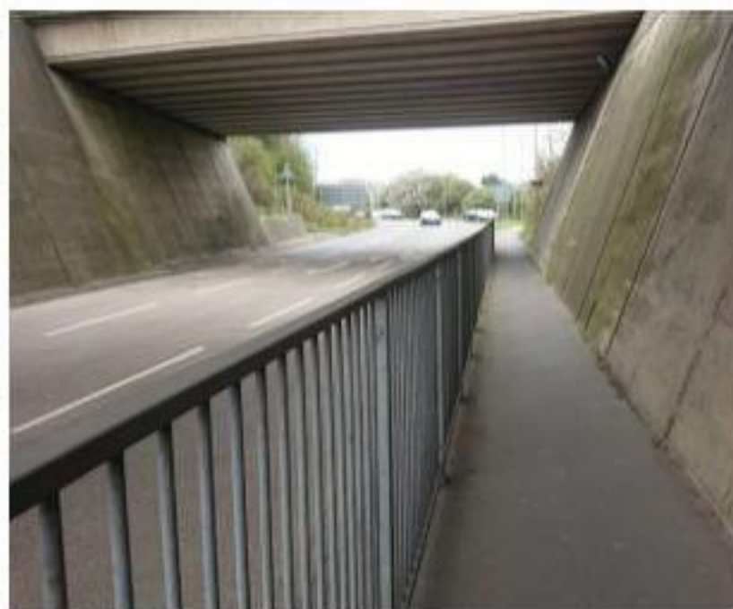
Photograph 7: Footway under A3M Motorway Bridge
