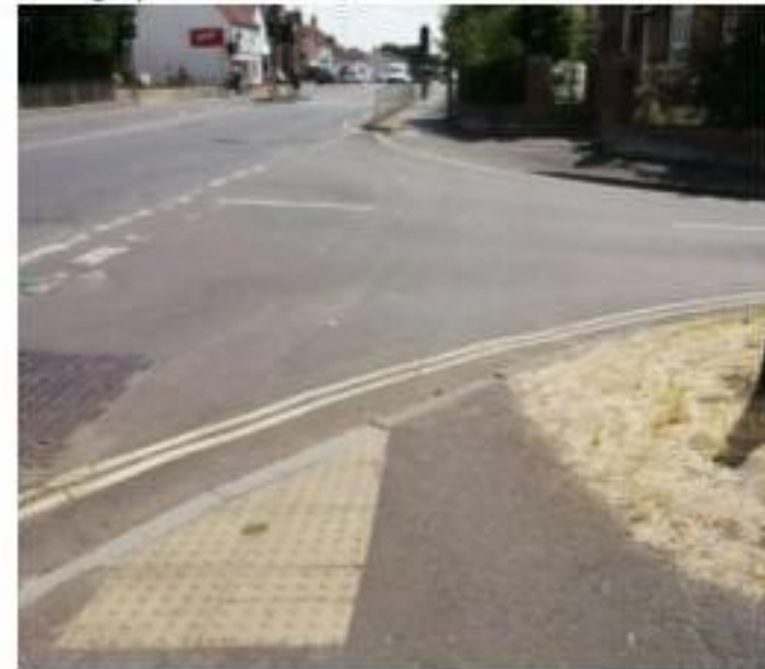
Photograph 44: Crossing at Kings Croft Lane
