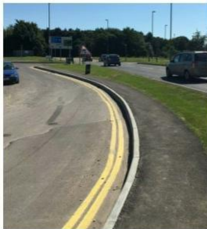
Photograph 3: Footway on Bedhampton Hill (Where footway/cycleway ceases)
