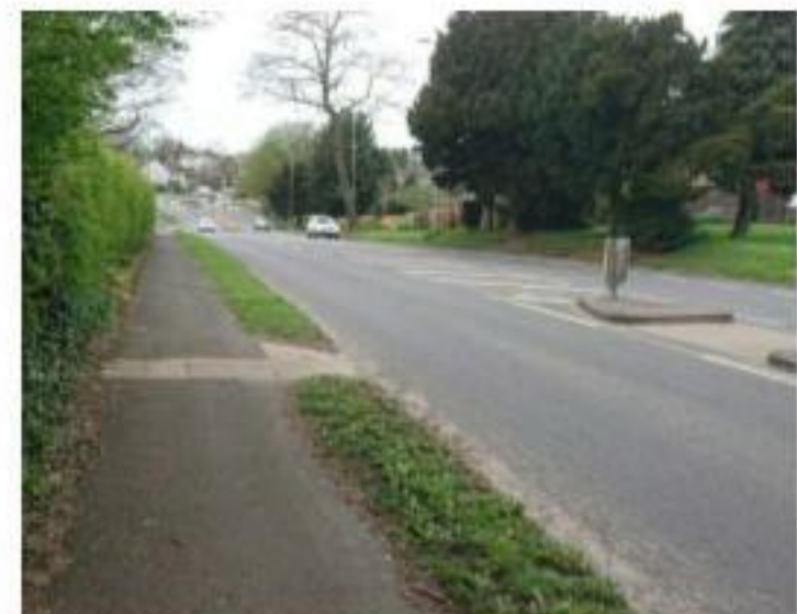
Photograph 47: Footway Conditions along Bedhampton Road
