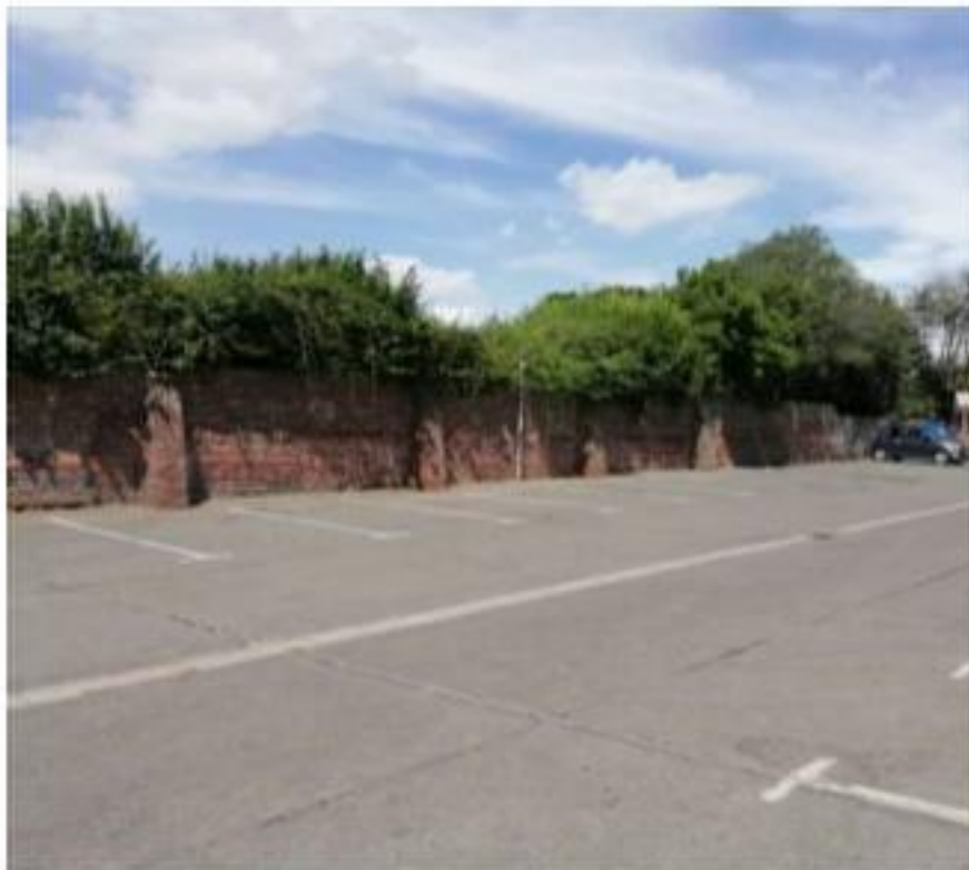
Photograph 57: Potential Park and Stride Site
