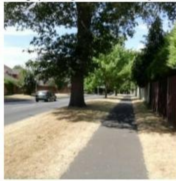
Photograph 64: Conditions along Emsworth Road
