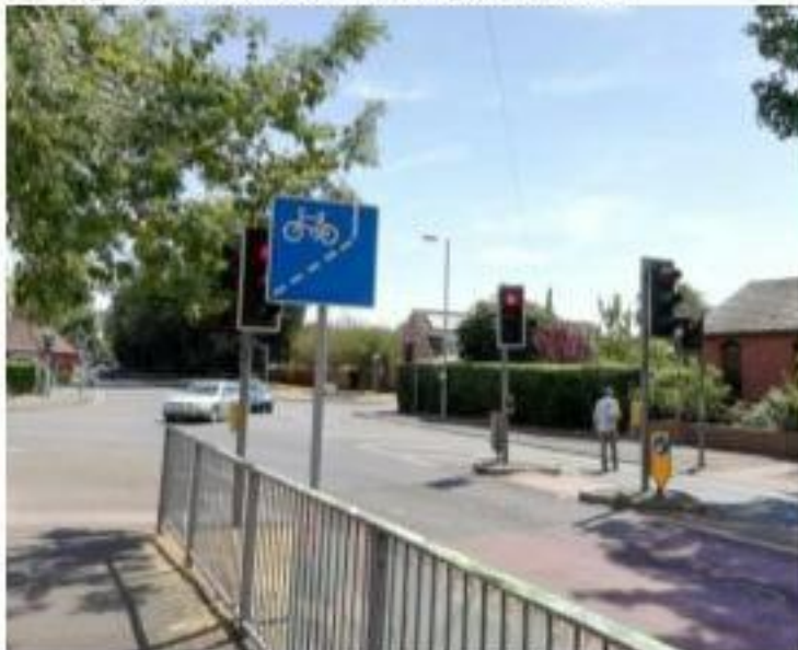
Photograph 65: Signal Control Crossing at Emsworth Road
