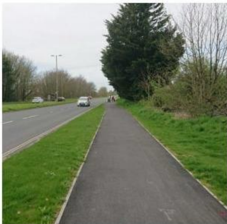
Photograph 2: New footway/cycleway along Havant Road
