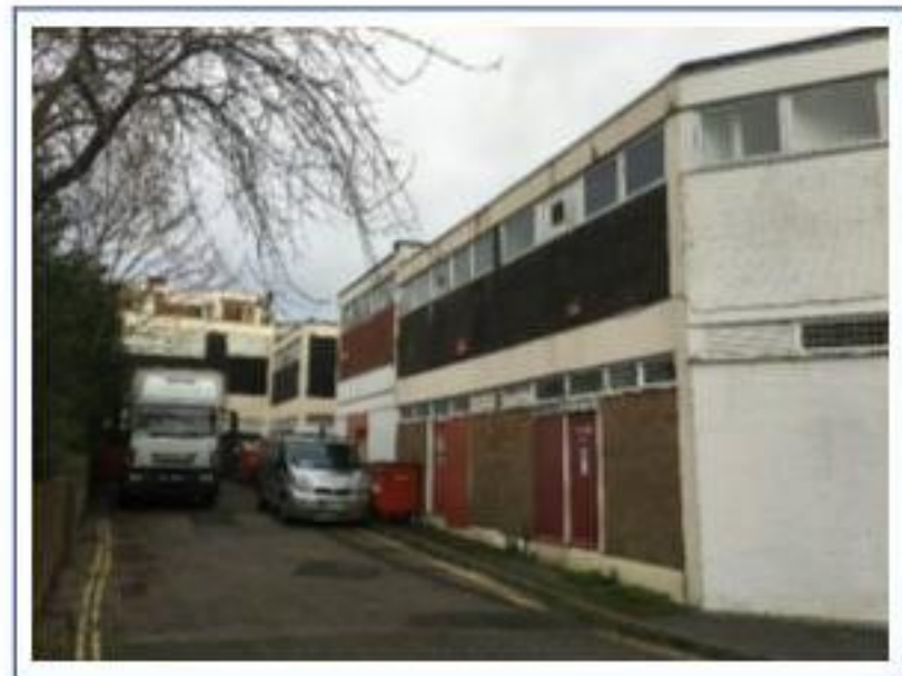
Tradesman entrance behind north western block
