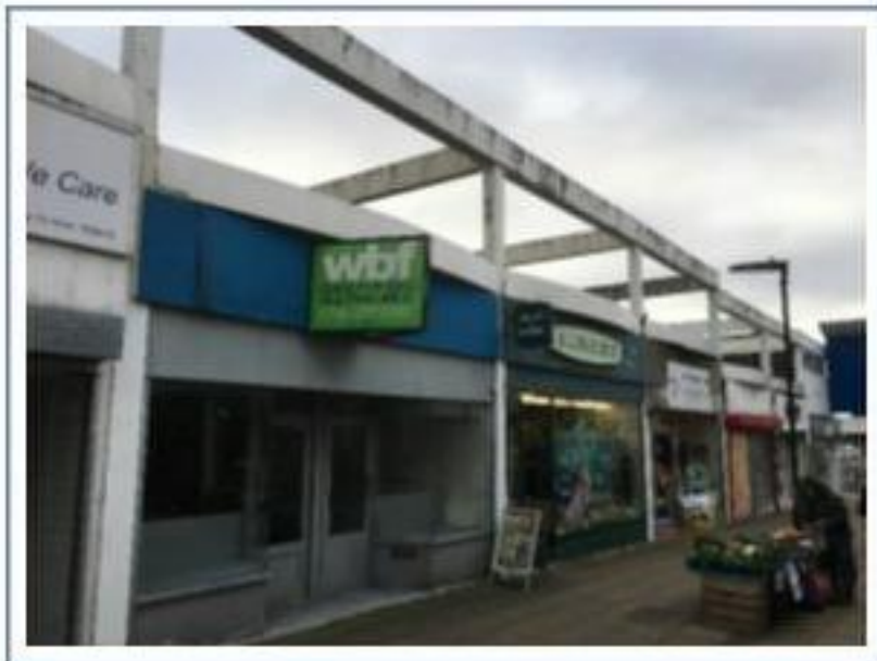
Retail units and view of concrete frame
