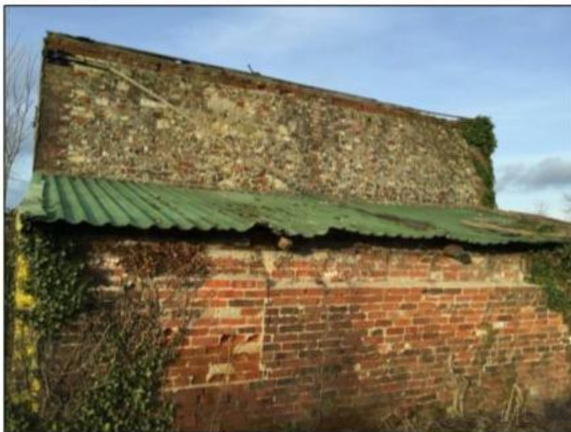
Photograph 21: Brick building located within the industrial area
