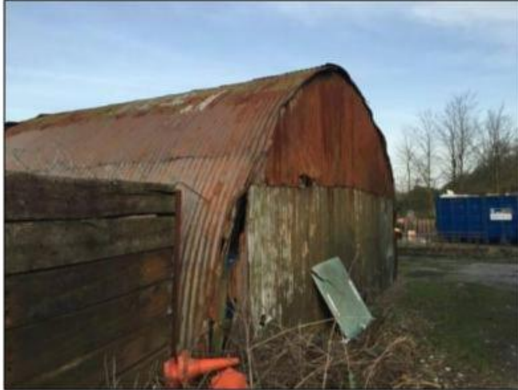
Photograph 20: A cylindrical roofed storage building located in the industrial area.
