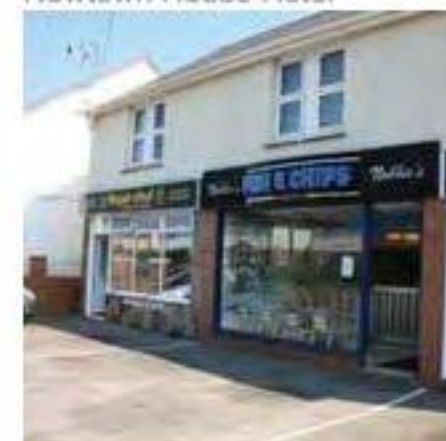
Facilities on Elm Grove
