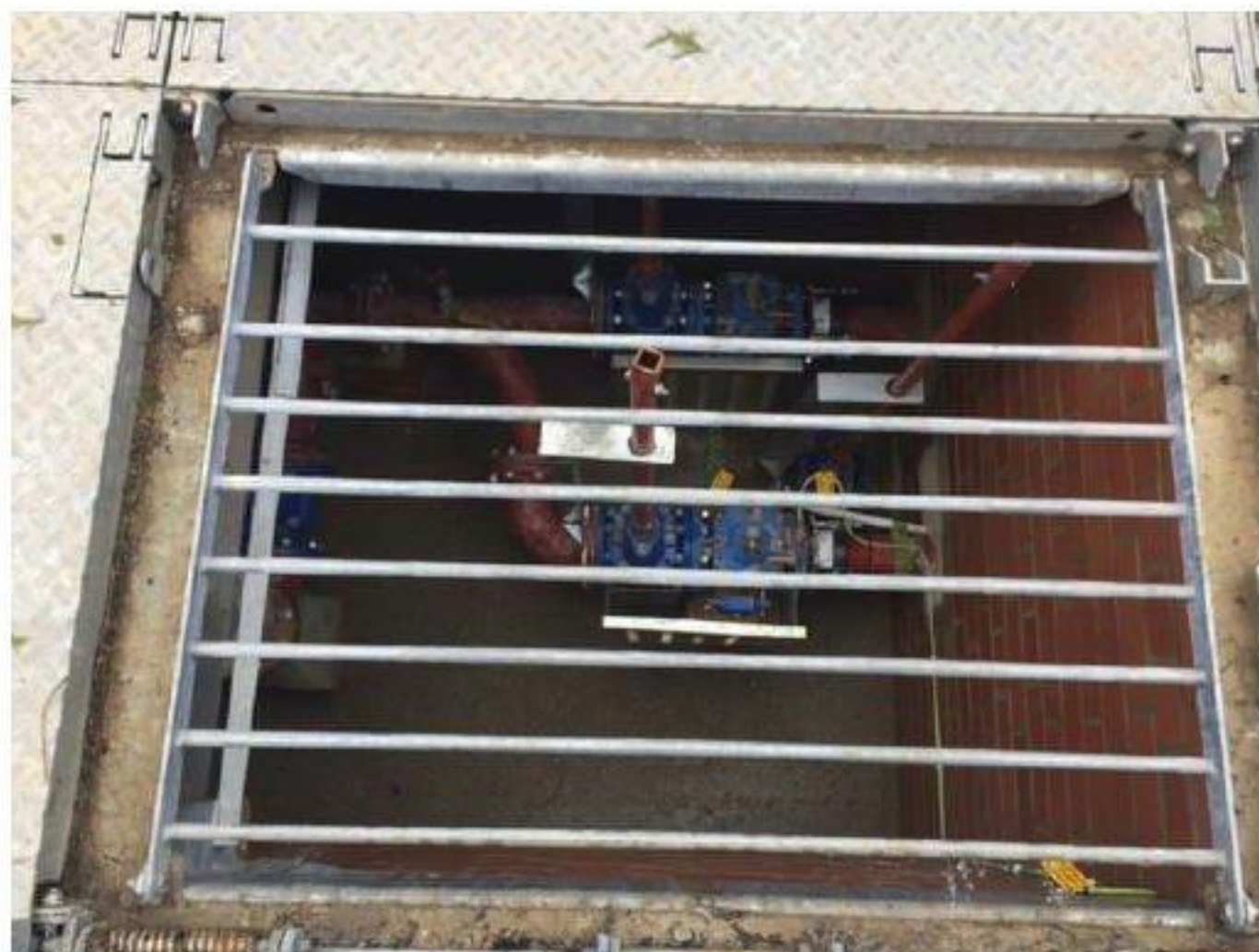
Cover removed over pumps during noise level monitoring
