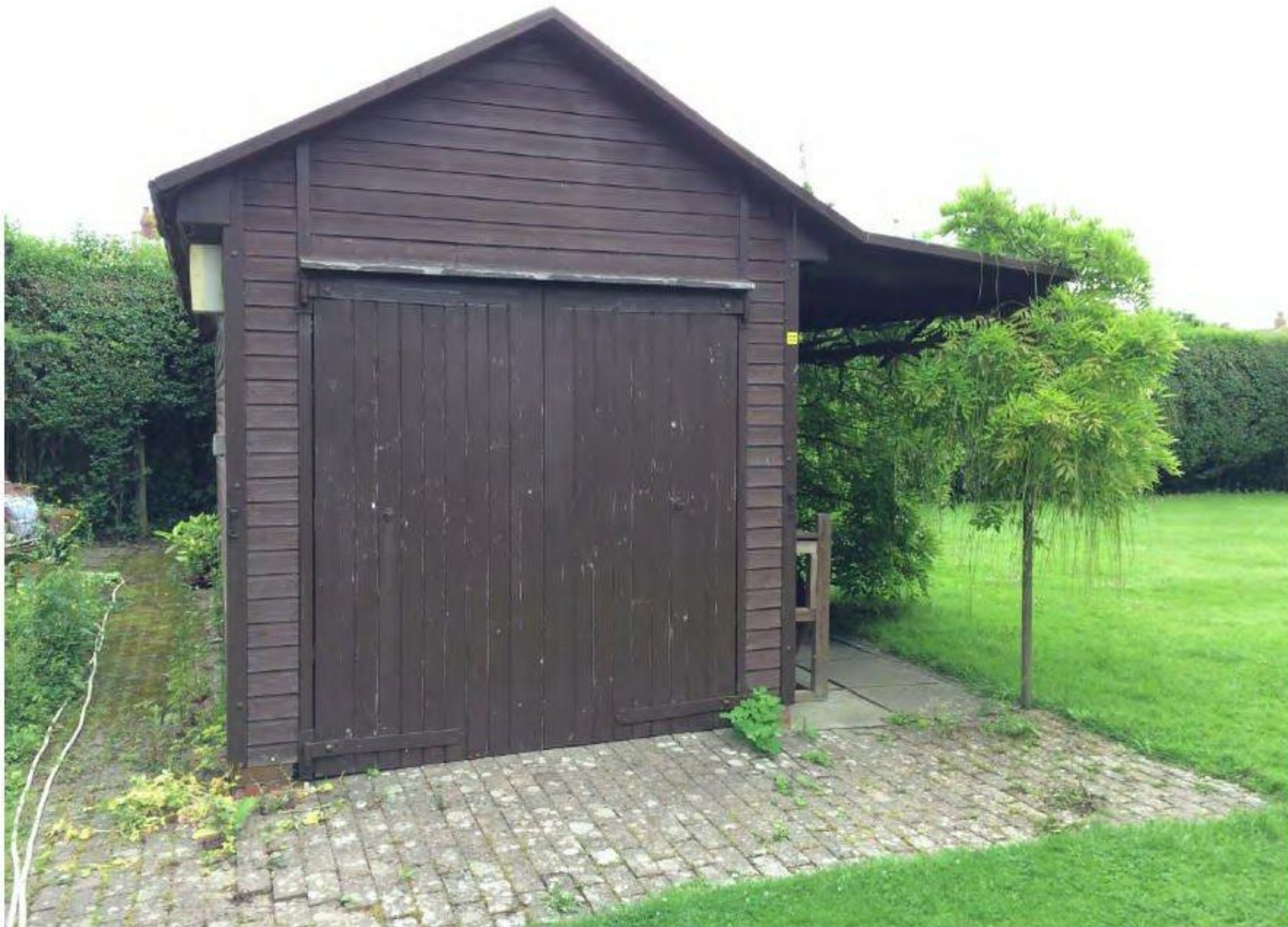
Plate 9. Timber Garden Store present in north-eastern corner of site.
