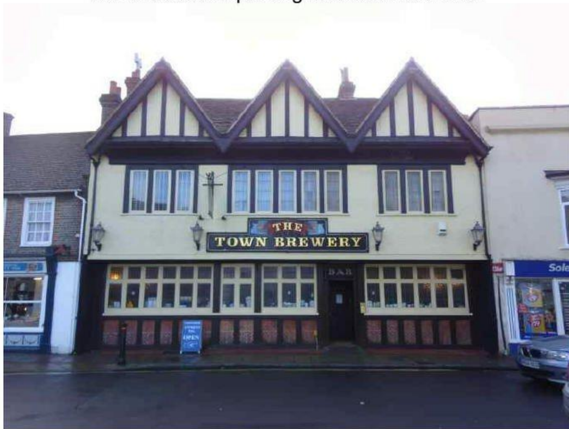
Fig 1: West Street elevation looking south.
