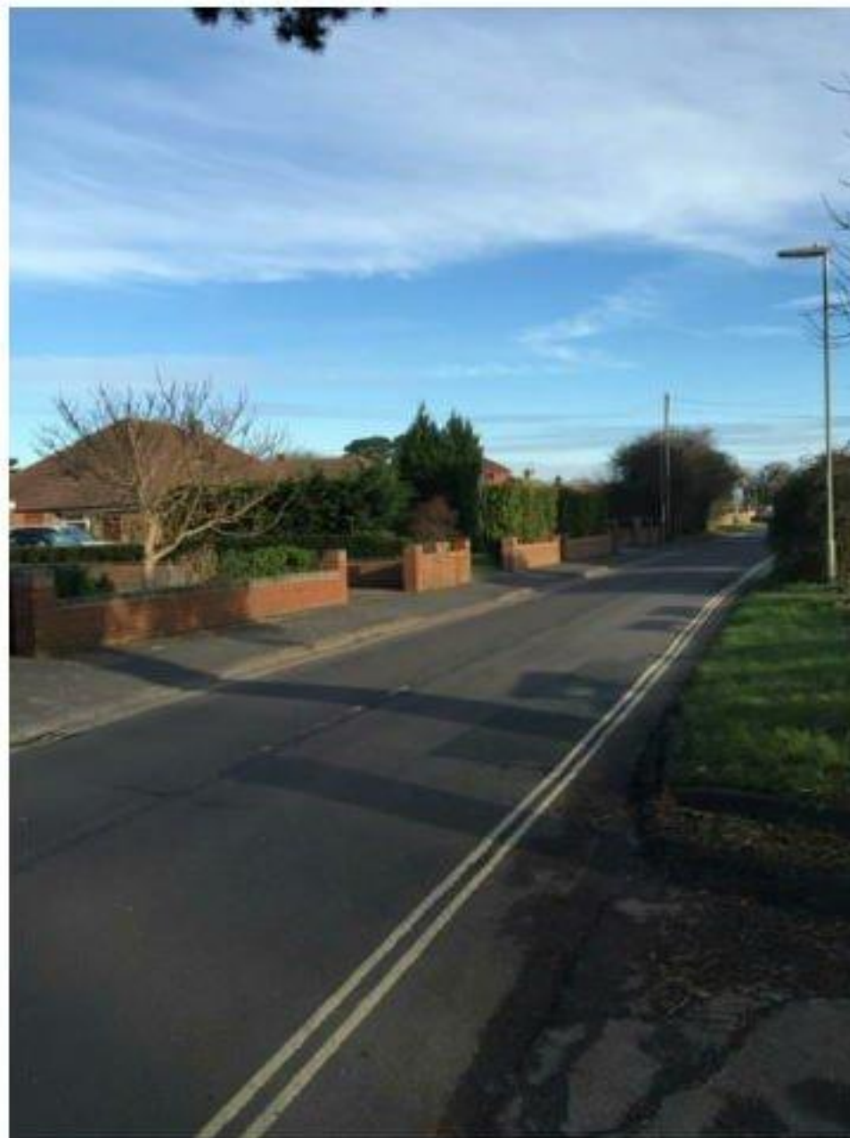
Photograph 1: Conditions on St Mary's Road
