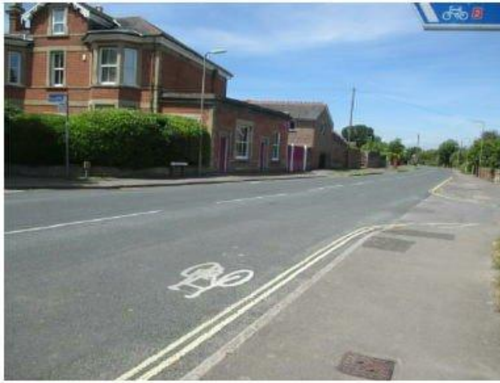
Photograph 4: Station Road on road cycle route
