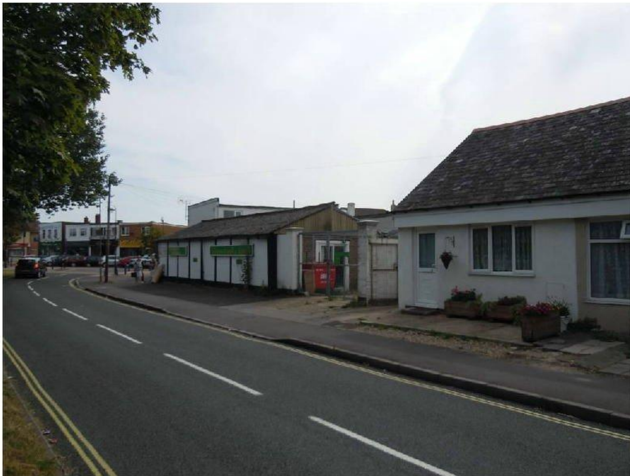
Side workshop from West Lane looking southwest
