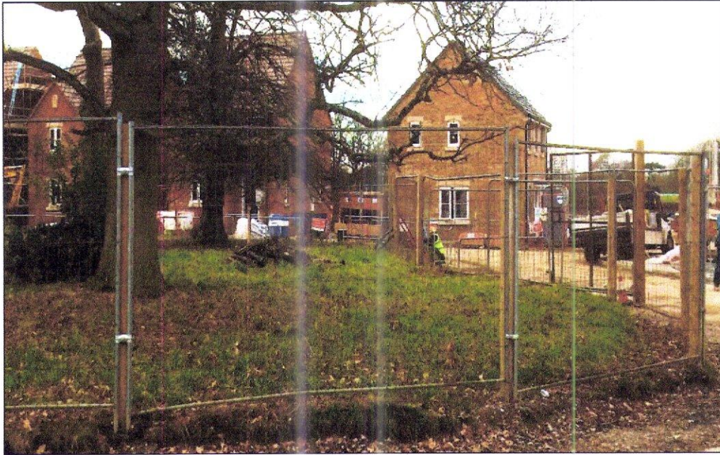
Weld-mesh panels on wooden posts
