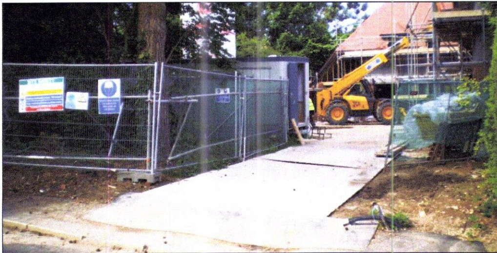
Vehicular ground protection trackway
