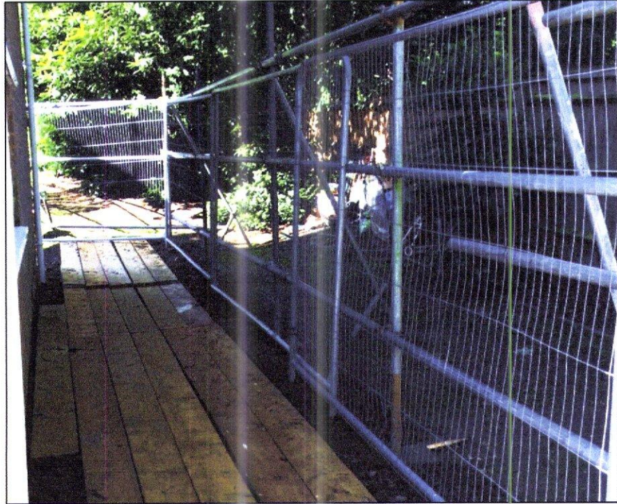
Scaffold board pedestrian ground protection
