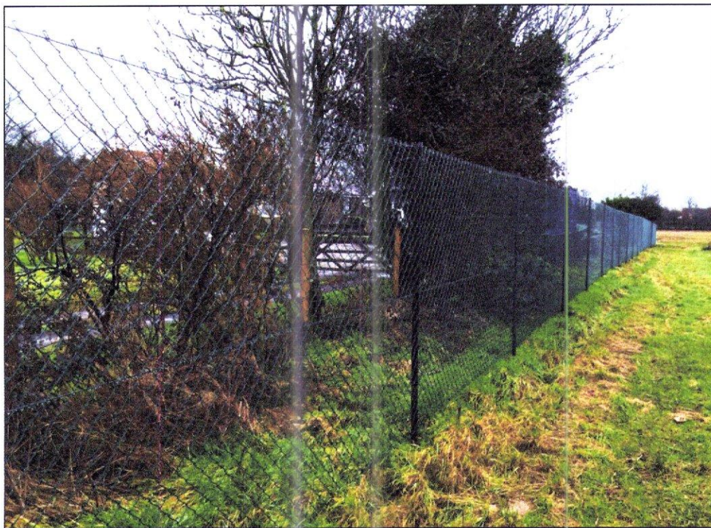
Chain-link on angle-iron uprights
