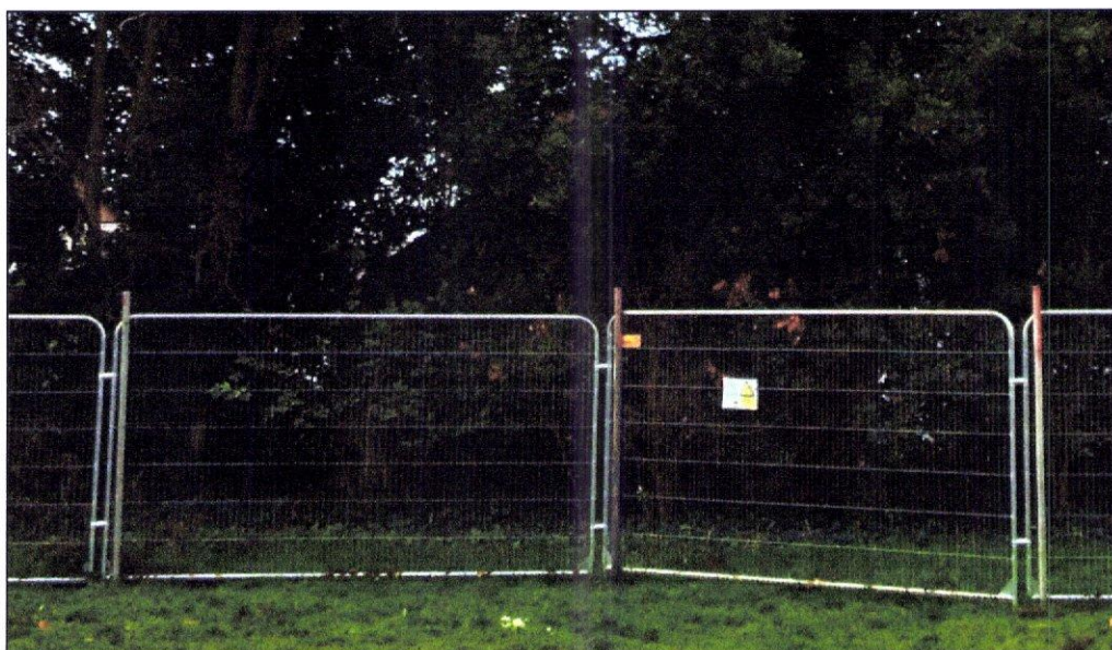
Weld-mesh panels on scaffold uprights
