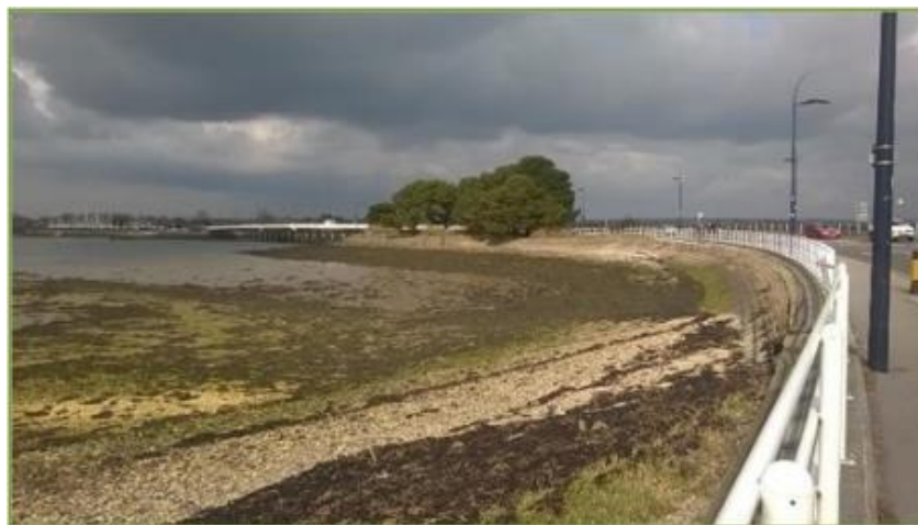
The A3023, connected by the Langstone Bridge from the mainland to the island.
