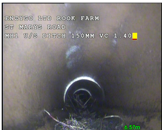
Photo: 3_3_18_A.jpg 6.57m, Roots, tap, Start
