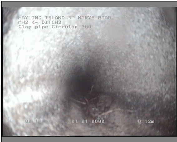
Photo: 1_1_4_A.JPG 0.12m, Material changes, concrete
