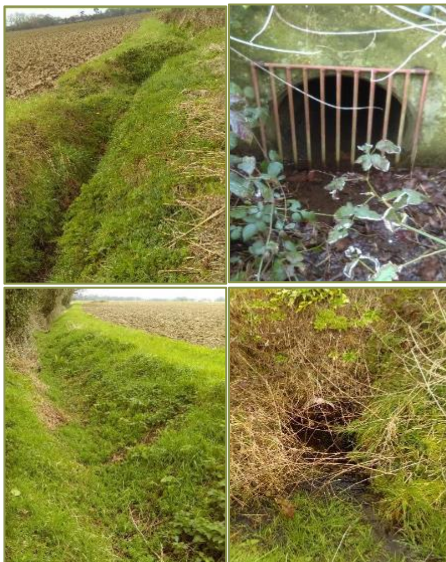
Top Left: Drain 4. Top Right: Drain 1 Ø450mm culvert outfall. Bottom Left: Drain 2 facing downstream. Bottom Right: Drain 3 looking downstream.
