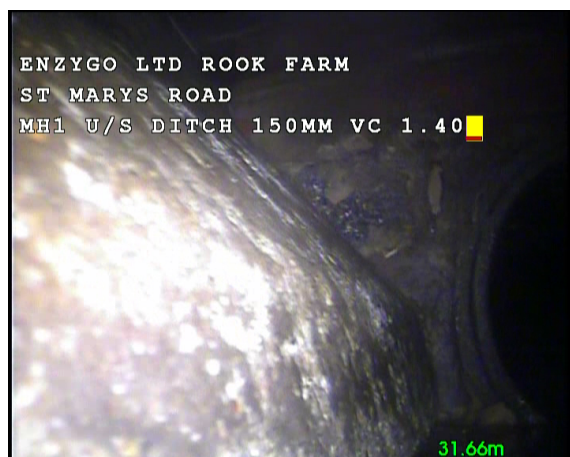
Photo: 3_3_22_A.jpg 31.66m, Finish node type, manhole reference number: U/S
