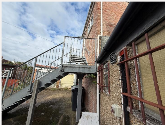
Staircase to rear of no 57.
