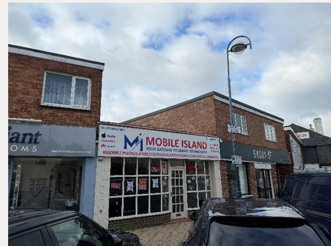
Existing shop front
