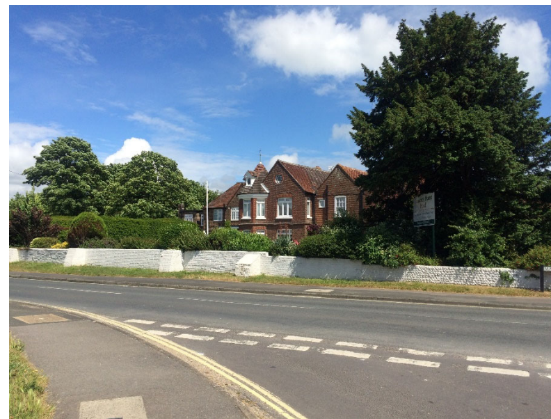
Plate 9: Newtown House Hotel as seen from the junction of Manor Road and Newtown Lane to the west.
