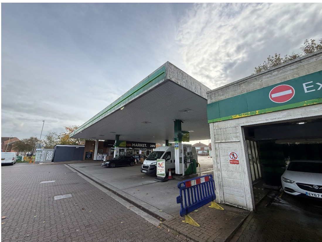
Photo 4: The majority of the Site is covered with paved brick, asphalt and concrete.
