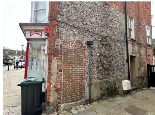
Flint on side elevation of 13A High Street, Emsworth
