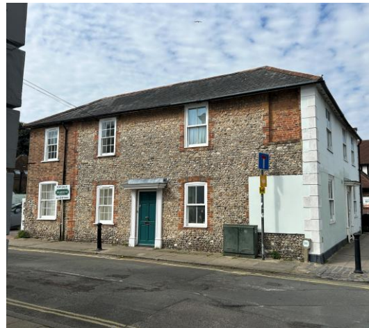
Flint on side elevation of 1 Tower Street, Emsworth
