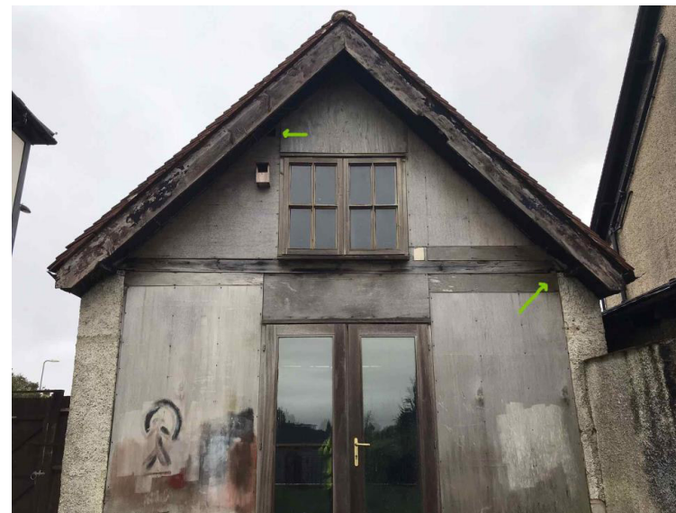
Plywood cladding to garage- Over clad with Hardie Plank. Replace existing timber windows and doors with UPVC
