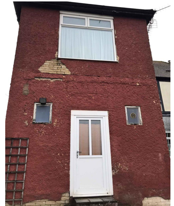
Timber windows replaced with UPVC.
