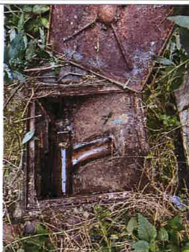
Manhole / Access Point: IC2 Internal
