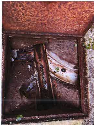
Manhole / Access Point: IC1 Internal
