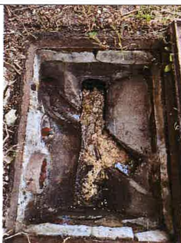
Manhole / Access Point: IC3 Internal
