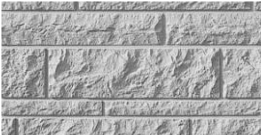
Imprinted concrete (blockwork effect)
