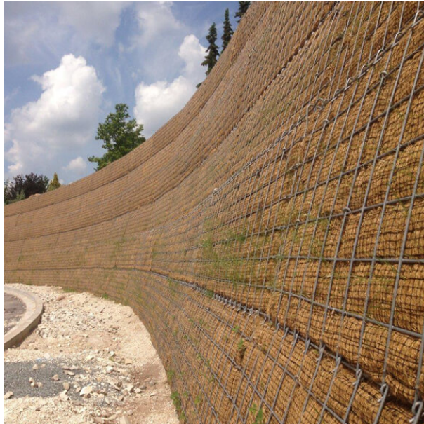
Figure 3a – Examples of TensarTech® GreenSlope System prior to planting with steel mesh facing and erosion control layer completed
