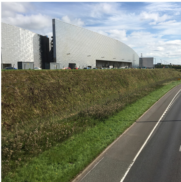
Figure 3b – Examples of fully vegetated TensarTech® GreenSlope System
