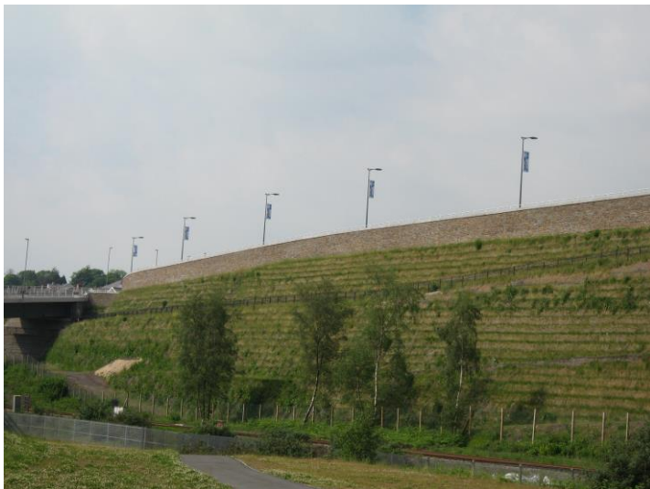
Figure 1. TensarTech GreenSlope for construction between 45 & 70 degrees
