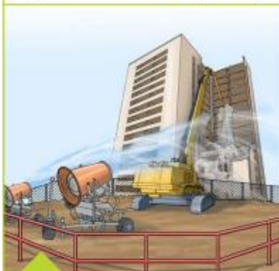
Long-reach 360 excavator munching a building.
