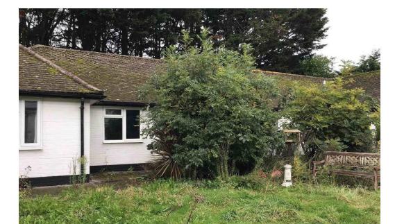
View of overgrown courtyard as existing
