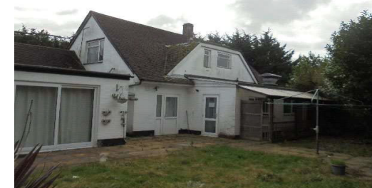
View of Rear Elevation
