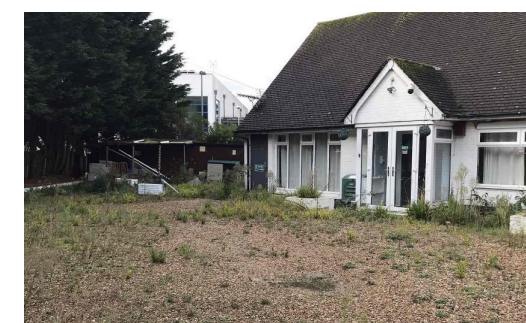
View of parking area as existing
