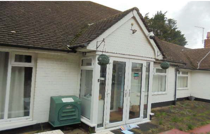
Existing gutters to be replaced and repairs to roof
