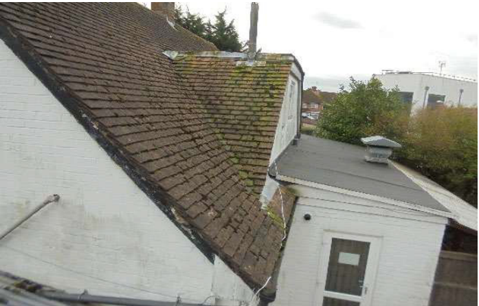
Existing roofs to be repaired/ replaced
