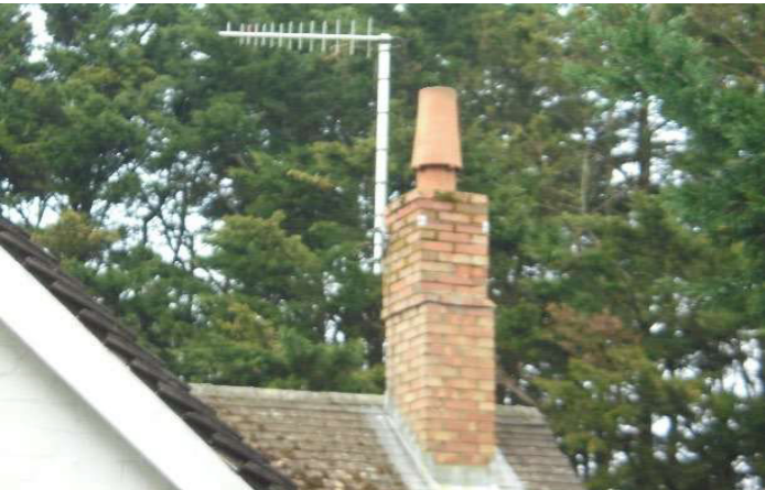
Existing Chimney to be re-pointed
