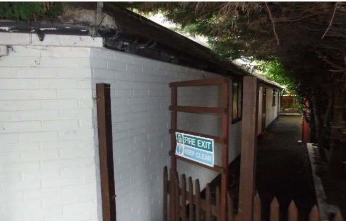
Existing gutters to be replaced and repairs to roof
