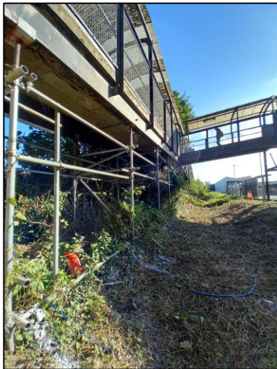
Photo 14 Existing ramps north of station.
