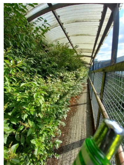
Photos 16 and 17 Foliage encroaching into currently closed ramp.
