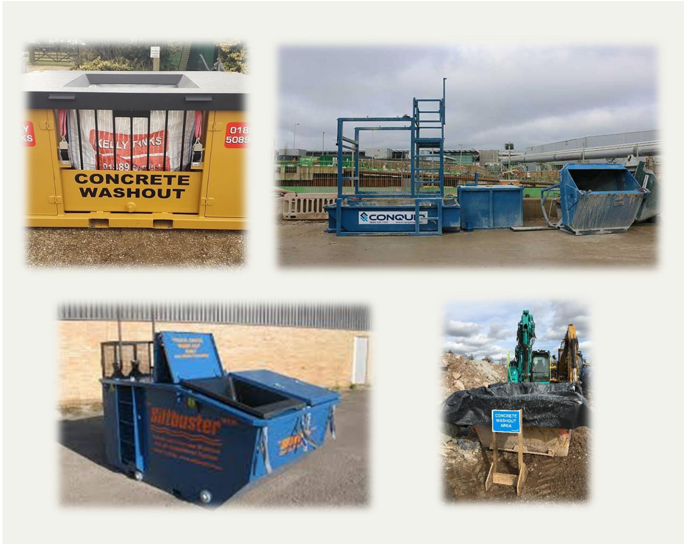
Figure 8 - Examples of Concrete Washout systems that may be utilised on site
