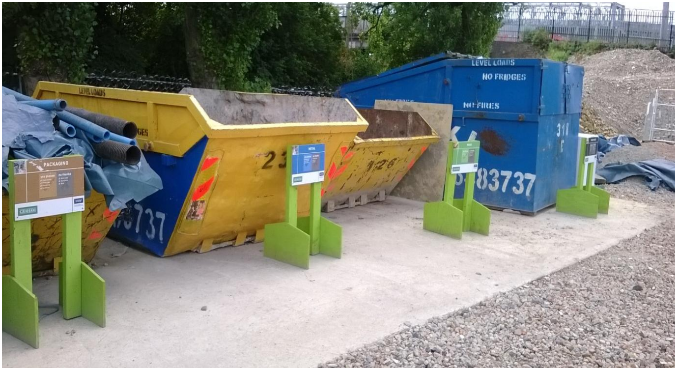
Figure 14: Waste Storage Arrangements
