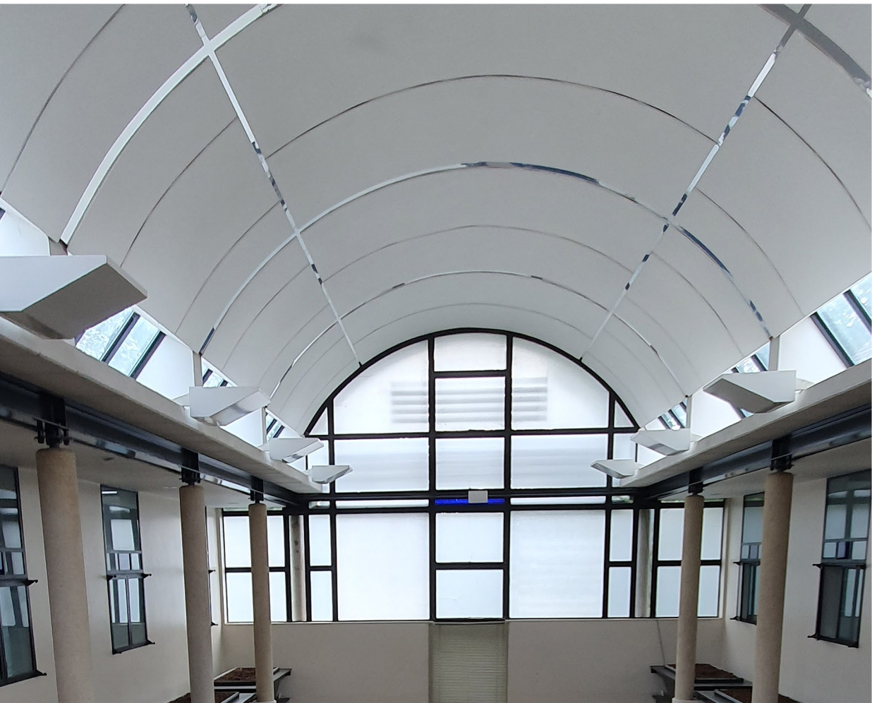
Existing photo of the rooflights above
