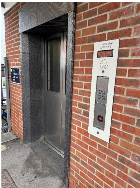
Figure 2-5: Lift at Station
