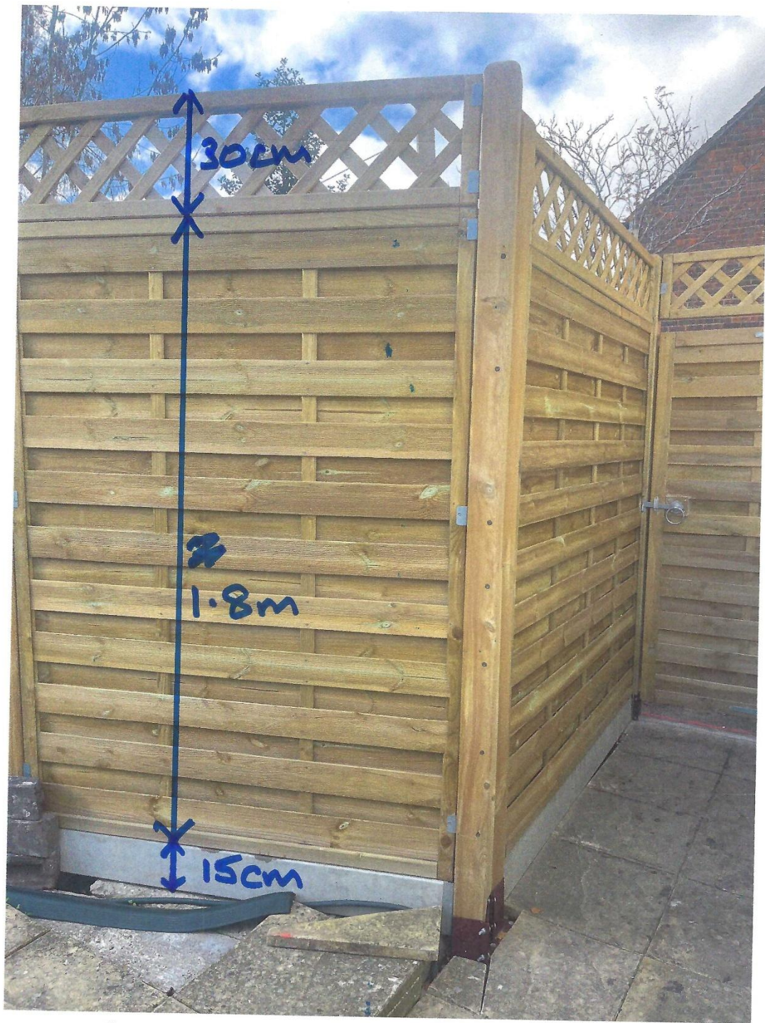
Shows fence + trellis + gravel board
