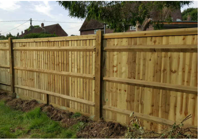
CLOSE BOARDED TIMBER FENCING
